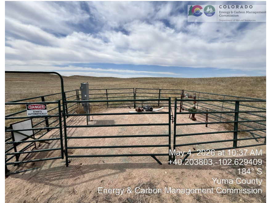
Unused equipment and Wellhead
