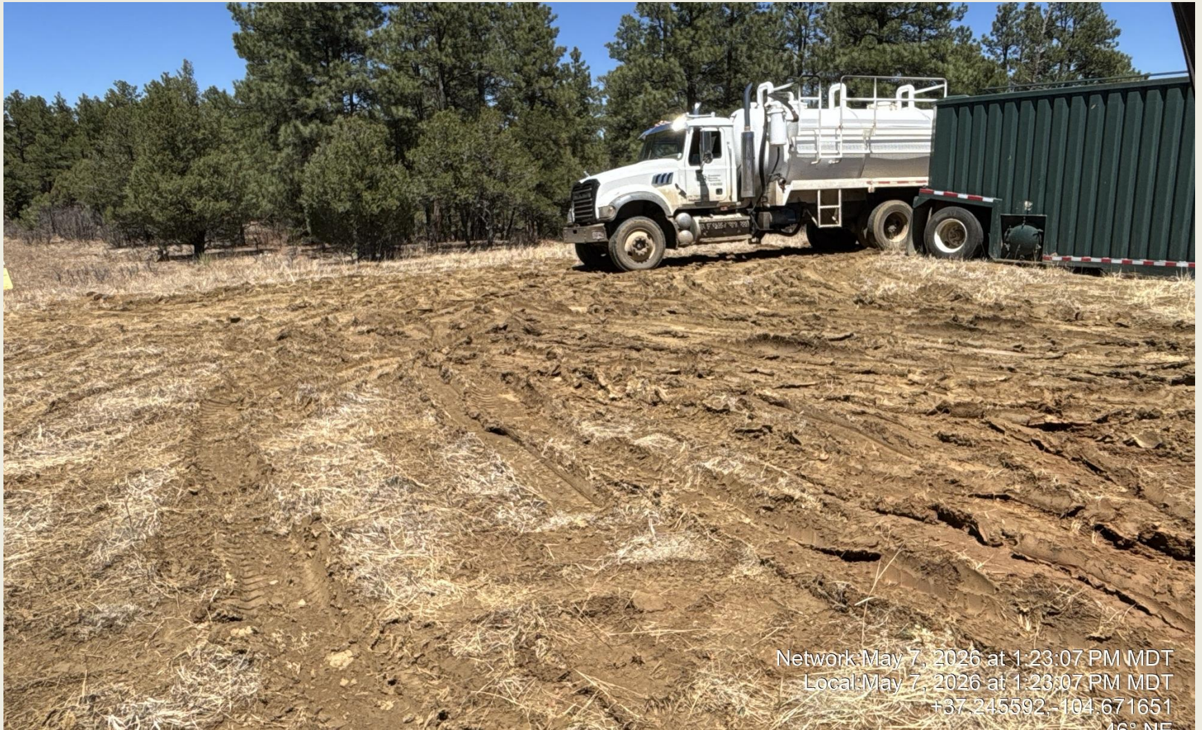
PHOTO 5: INTERIM RECLIMATION AREA WEST OF WELLHEAD WILL NEED RE-SEEDED. RE-SEED ALL DISTURBED INTERIM RECLIMATION AREAS PER RULE 1003. CA DATE 7/15/2026.
