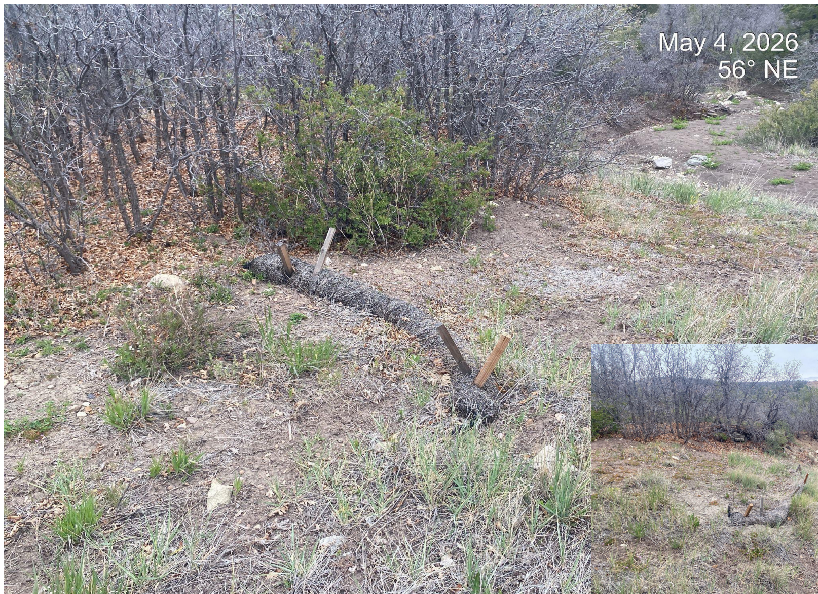
Photo 3. View of temporary plastic wrapped wattle BMPs which remain at the reclaimed well pad access point.
