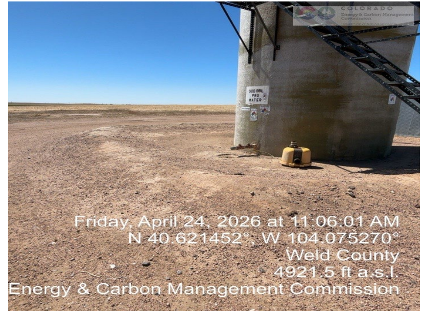
Photo 4 – Tank Berms inadequate
