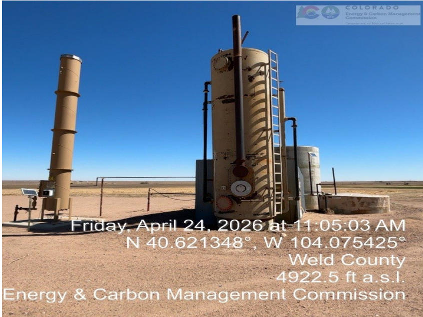
Photo 1 – Heater Treater and ECD
