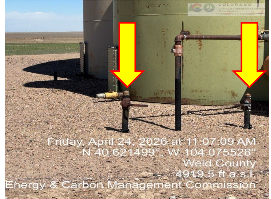
Photo 8 – Unmarked Risers
