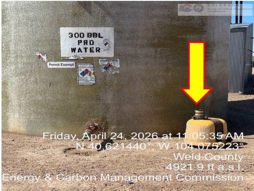
Photo 3 – Tank Labels – Unused Loadline Bucker
