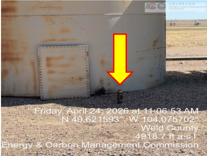
Photo 7 – Unmarked Riser
