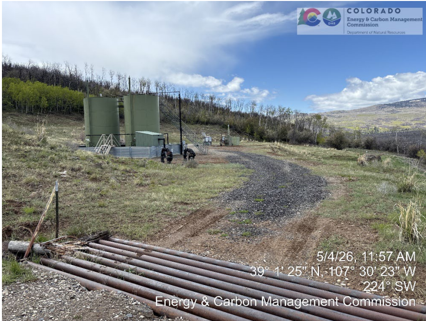
Location overview looking SW
