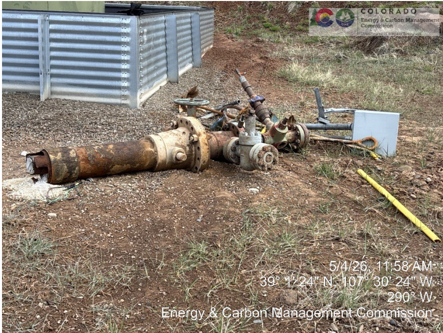
Cut off wellhead and valves
