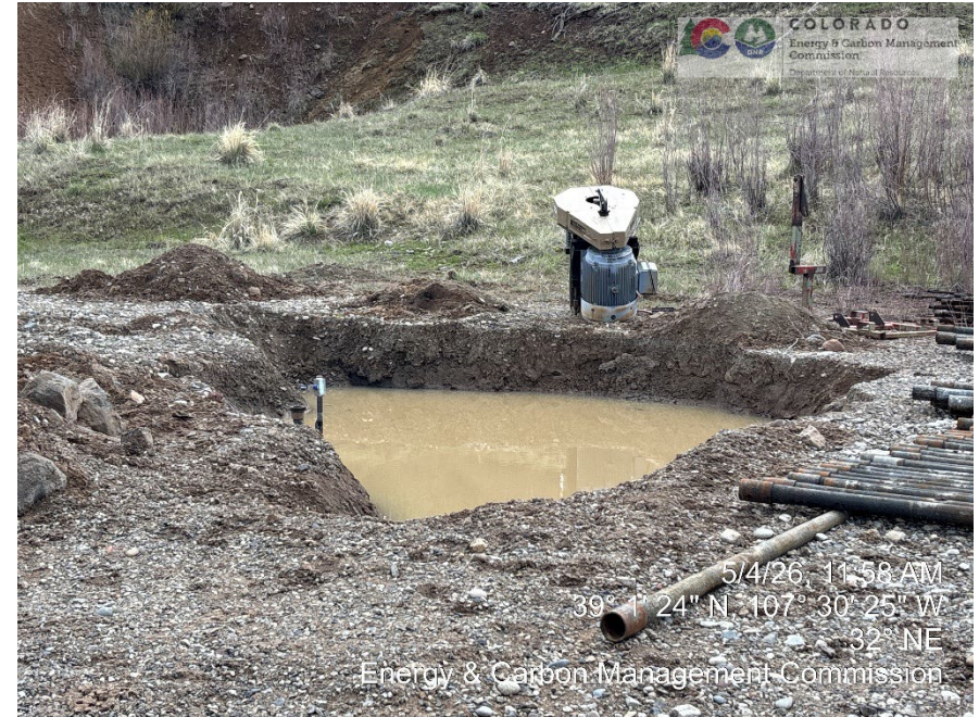
Excavations for Plugged and Abandoned well.
