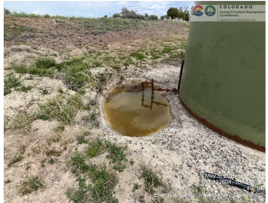
POSSIBLE FLOW LINE LEAK
