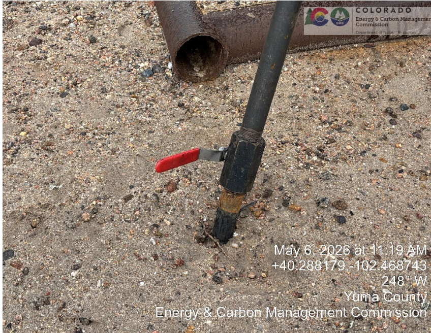
New water ground valve
