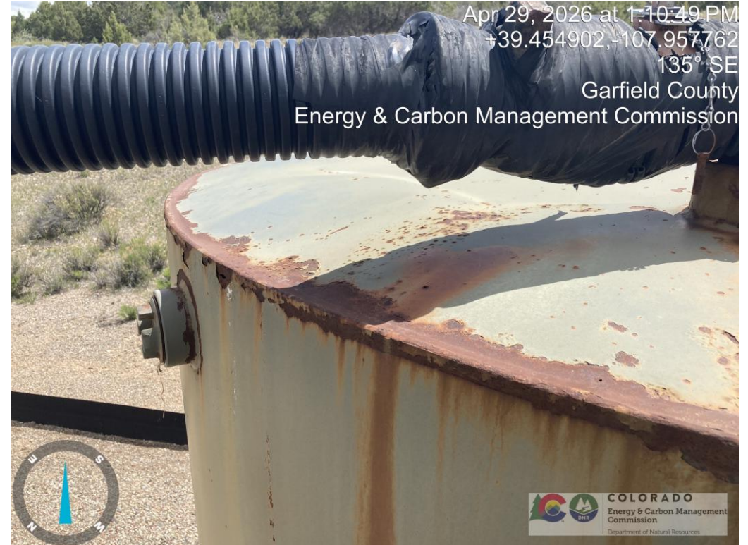
Rusted pin holes on top of tank.
