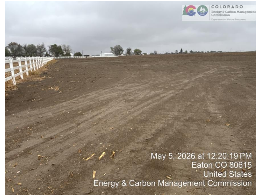
Photo 2 well site remediation area
