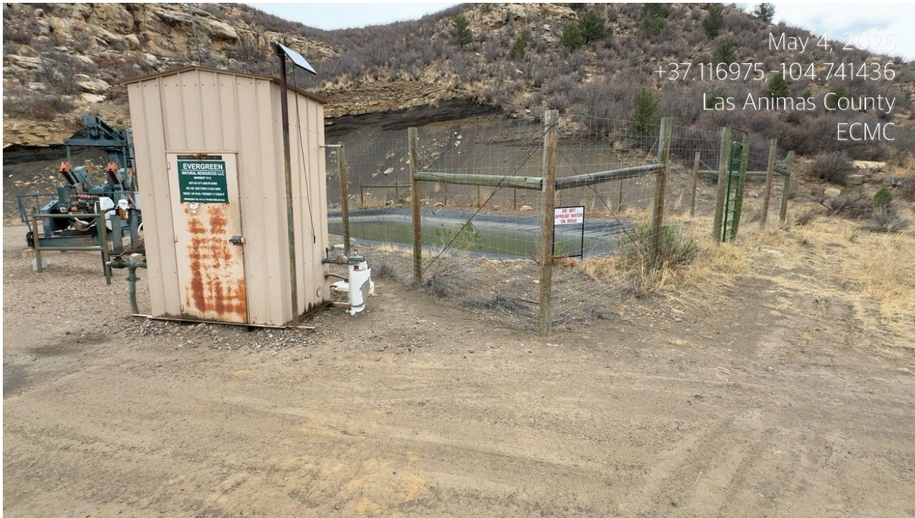
Photo 2. Facing toward the lined produced water pit.
