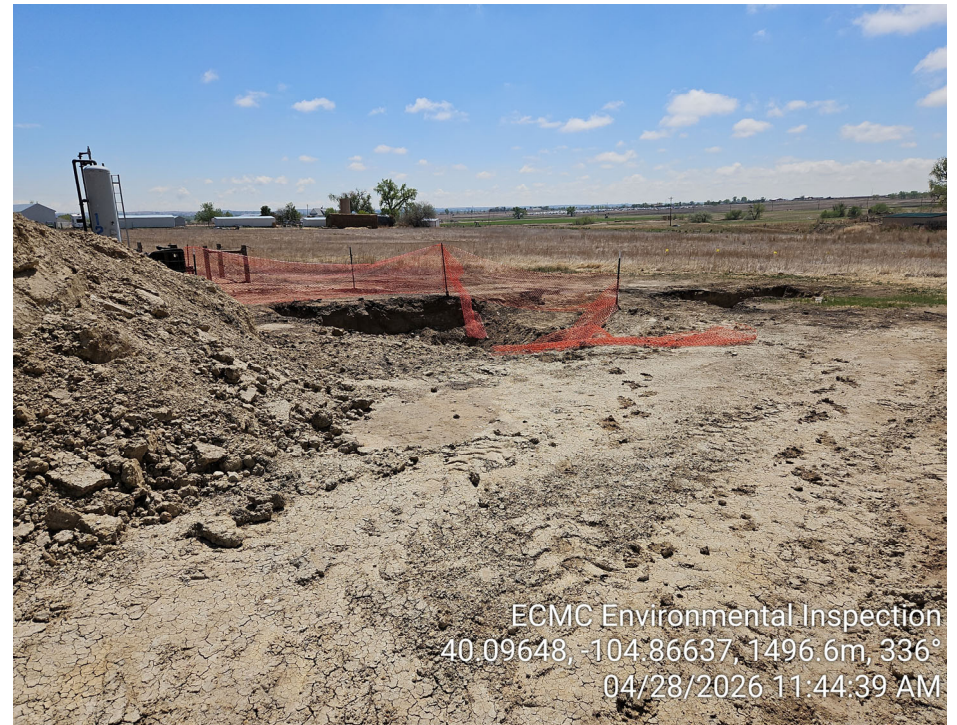
Photo 2 – Fencing down around open excavation. Soil stockpile with no liner or stormwater BMPs.
