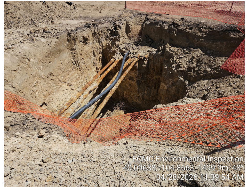
Photo 4 – Open excavation. Flowlines running through open excavation. Uncapped flowlines sticking out of excavation sidewall.
