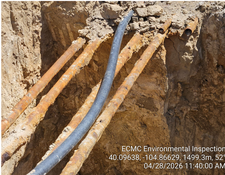
Photo 5 –Flowlines running through open excavation. Uncapped flowlines sticking out of excavation sidewall.
