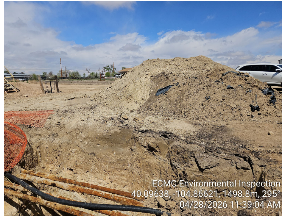
Photo 6 – Soil stockpile with no liner or stormwater BMPs.
