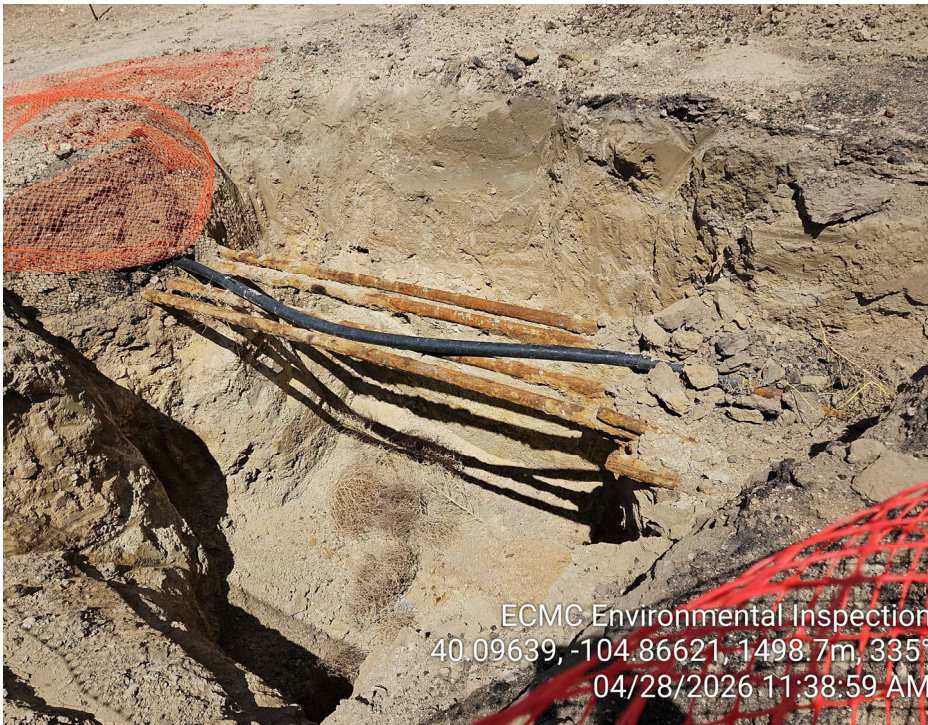
Photo 3 – Open excavation. Flowlines running through open excavation. Uncapped flowlines sticking out of excavation sidewall.
