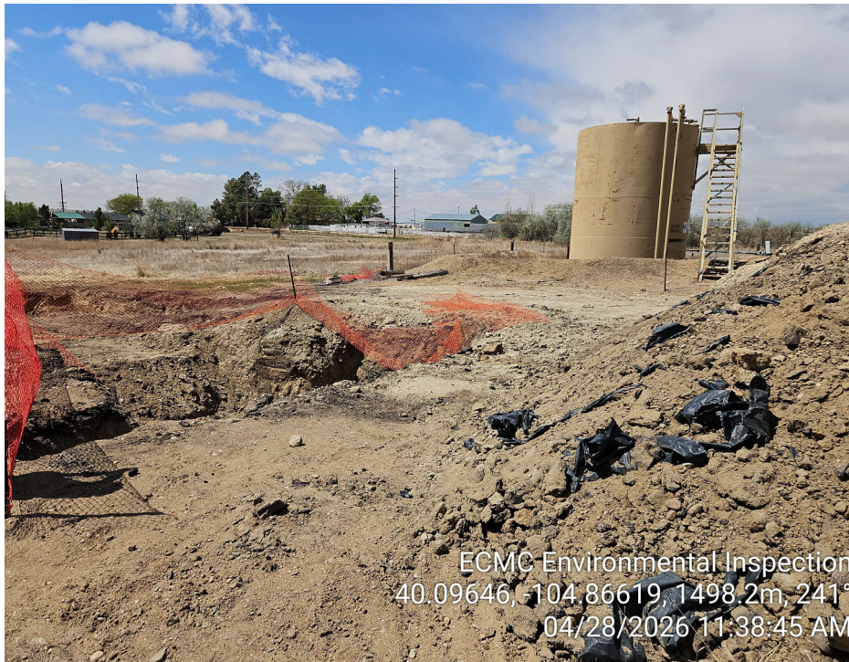
Photo 1 – Fencing down around open excavation. Soil stockpile with no liner or stormwater BMPs.
