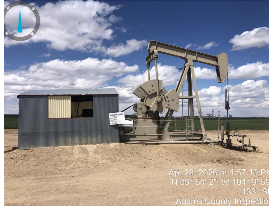
Photo #4 Pump jack.
