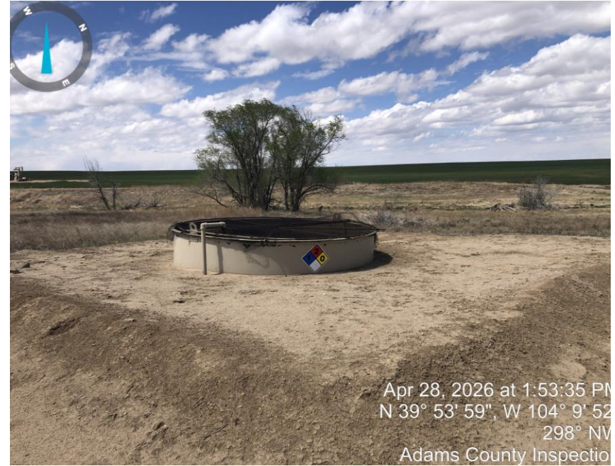
Photo #2 P/W tank.
