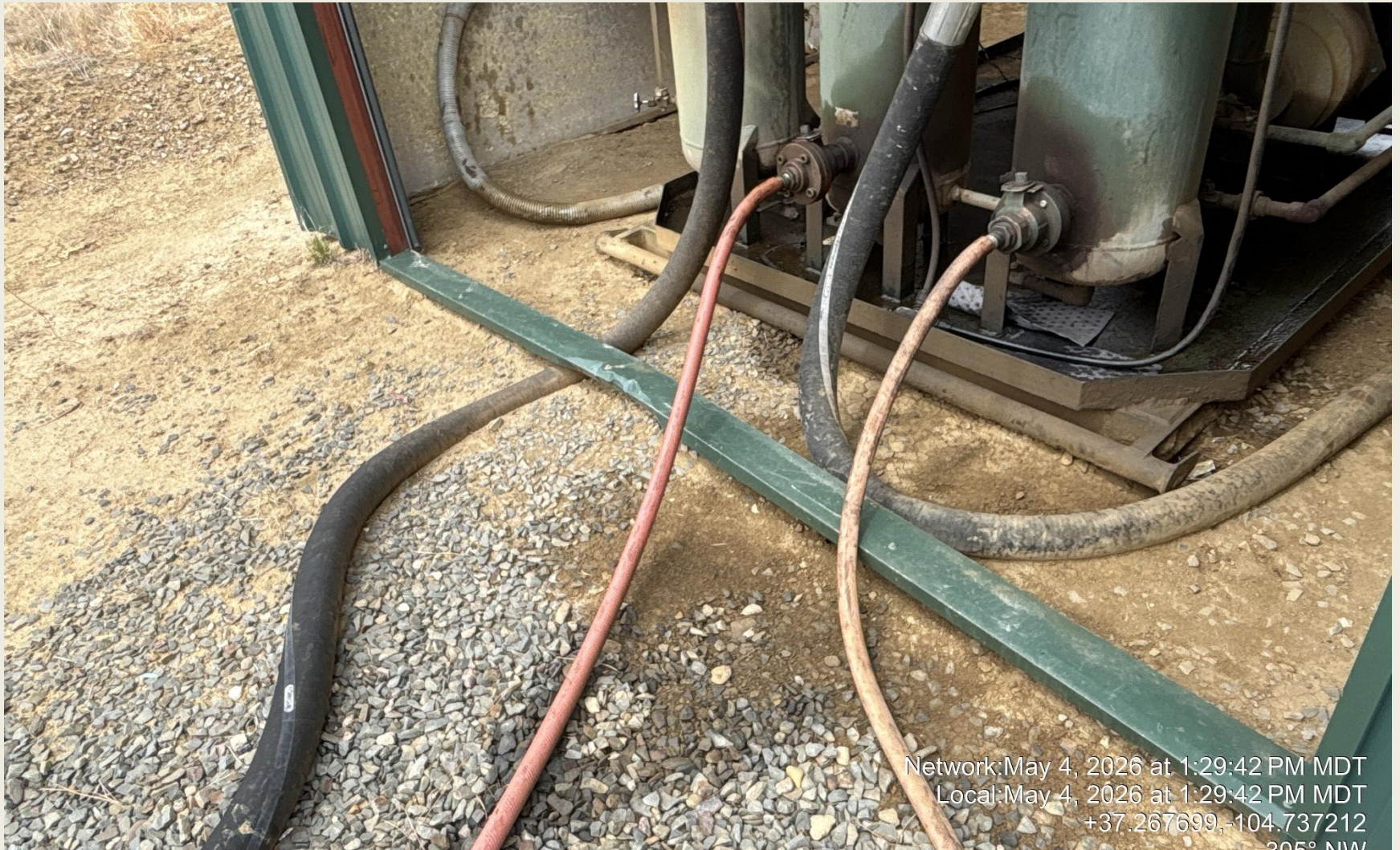
PHOTO 7: AREA OF IMPACTED SOIL NEAR TR WELL COMPRESSOR. Conduct maintenance on equipment, cleanup stained material and review self inspection processes. COMPLY WITH RULE 1002,(2).D. CA DATE 6/4/2026.
