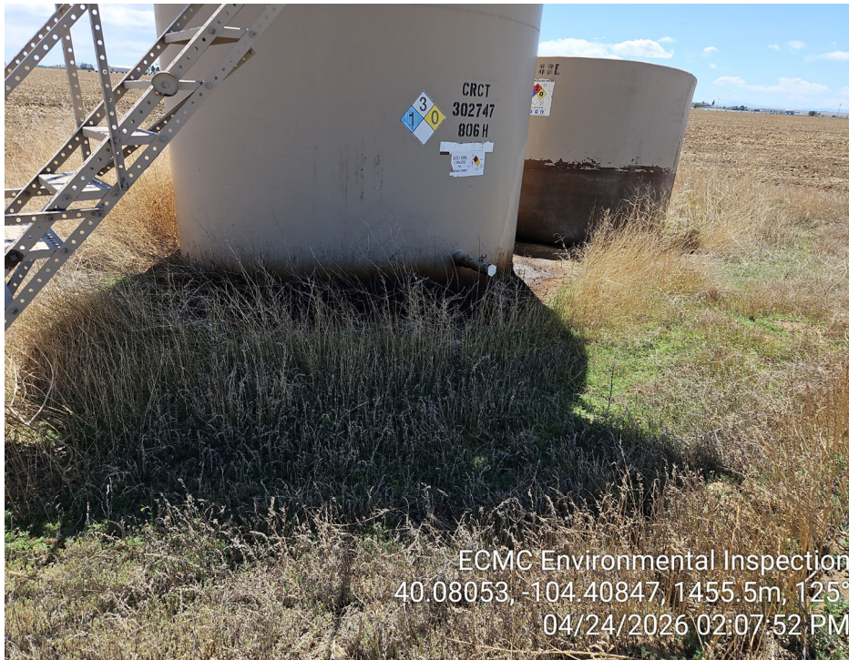
Photo 5 – Spill observed around AST
