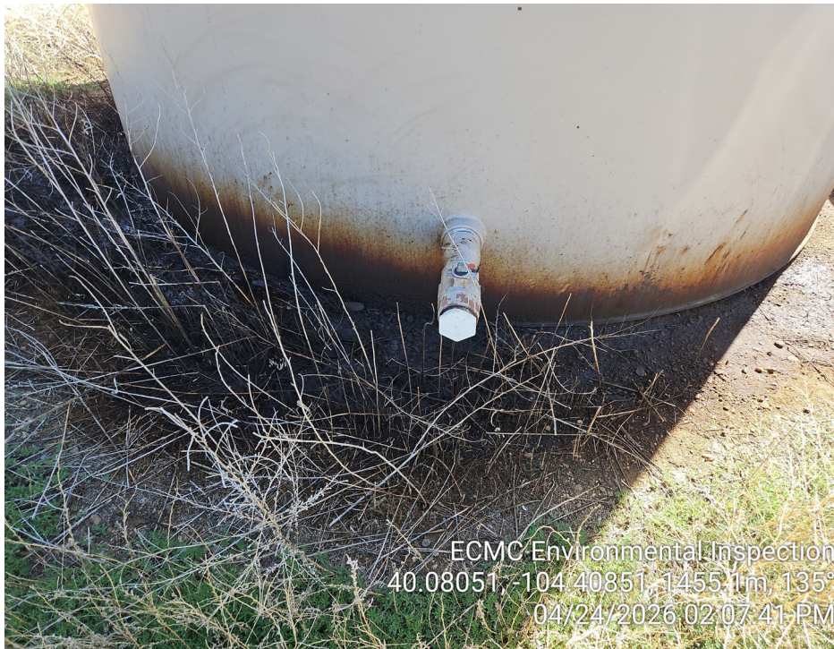
Photo 3 – Spill observed around AST
