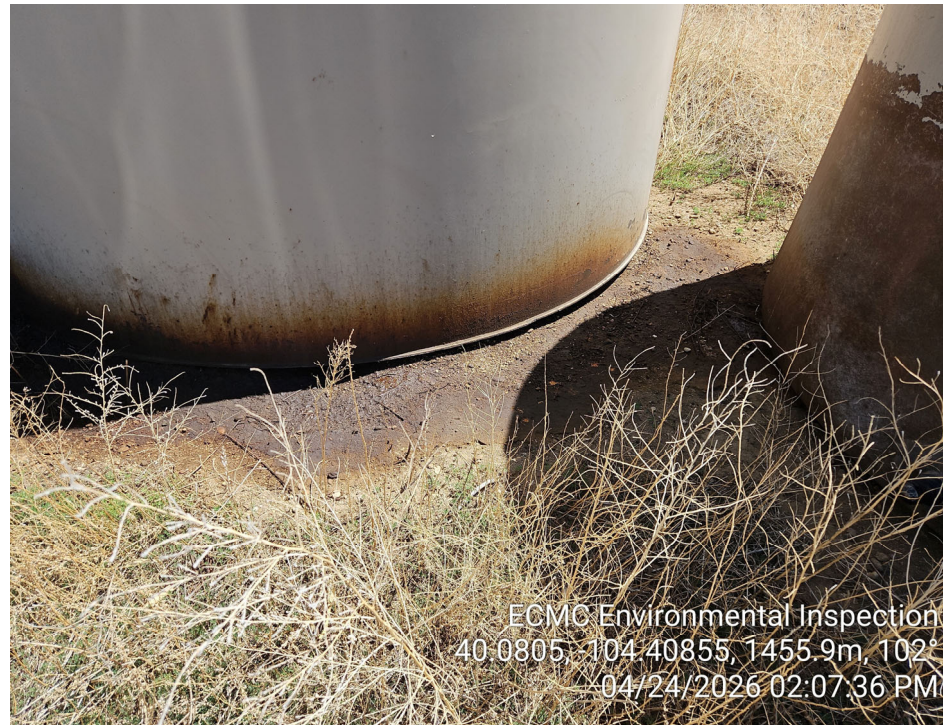
Photo 4 – Spill observed around AST
