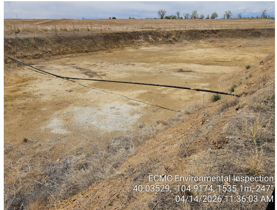
Photo 2 – Flowline Running through open excavation. Weeds on excavation sidewalls.
