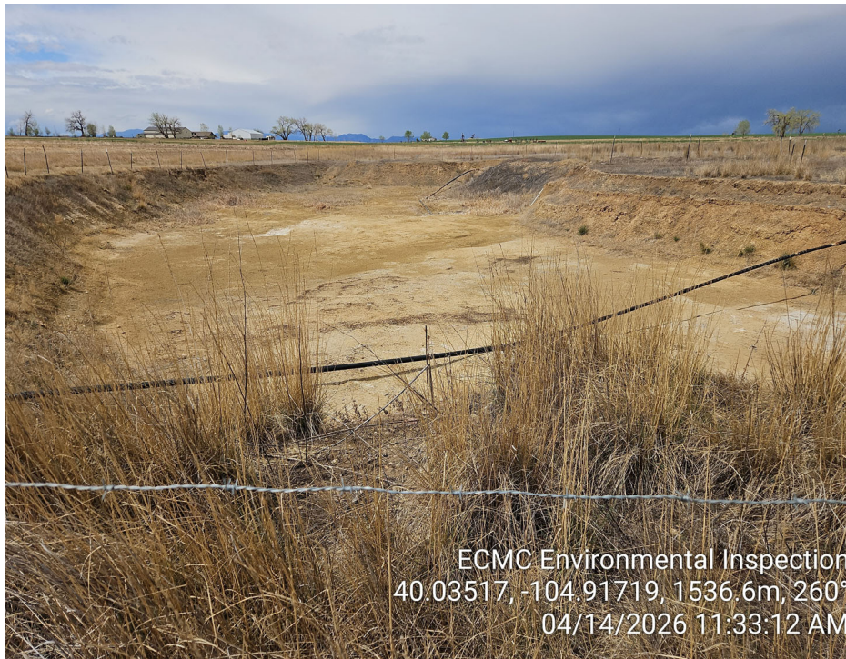
Photo 1 – Open excavation. Flowline runs through open excavation. No groundwater present. Weeds on excavation sidewalls.
