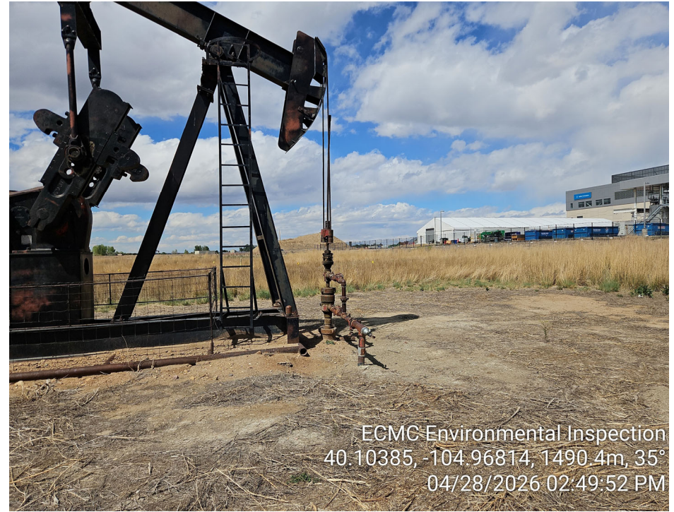
Photo 8 – Excavation previously observed at wellhead has been backfilled.
