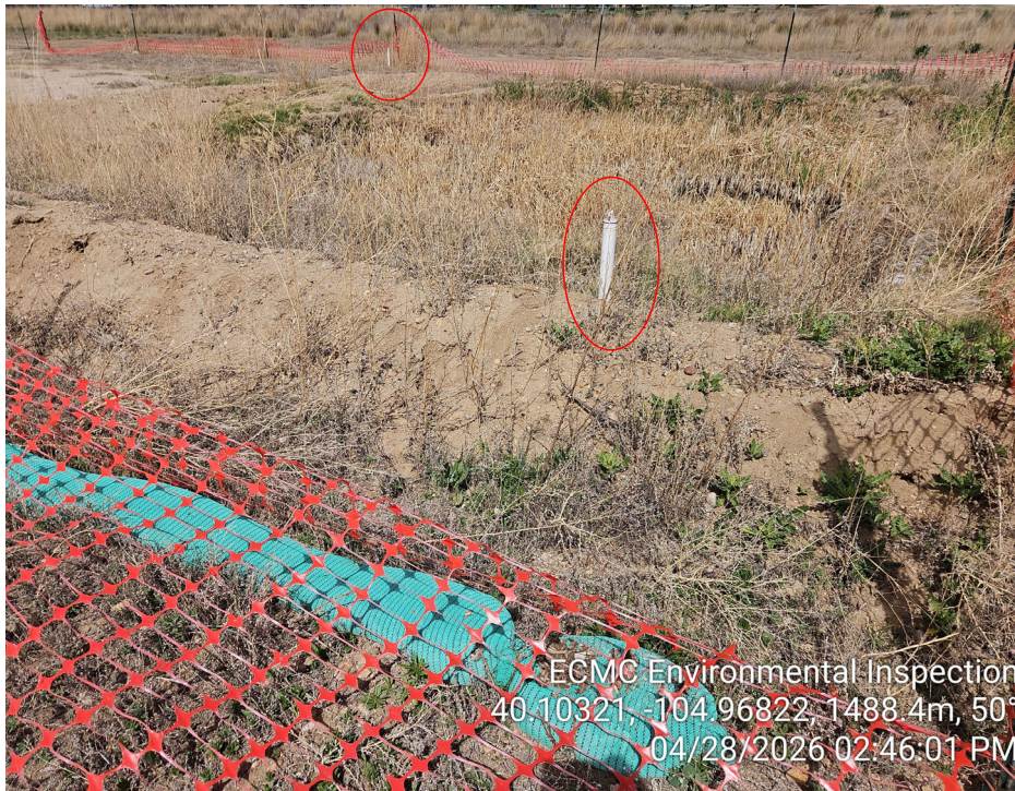
Photo 3 – Fencing down around open excavation. Stormwater waddles have degraded and become trash. Monitoring wells present around open excavation (red).
