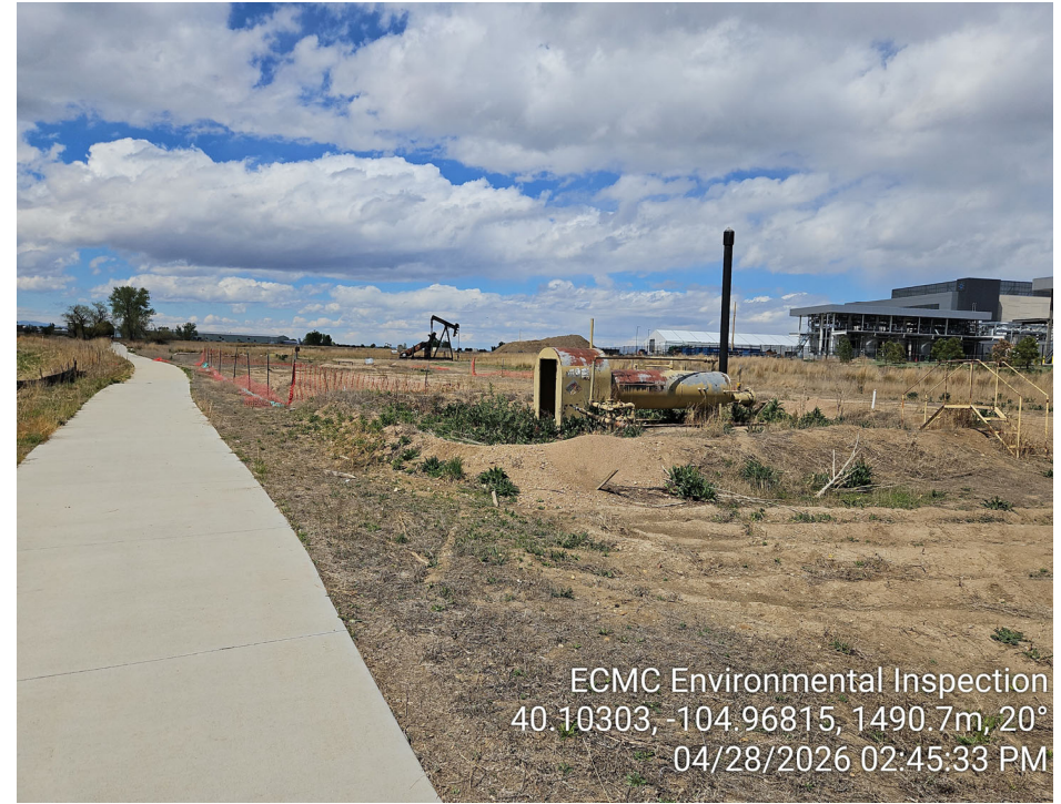
Photo 2 – Spill area. Fencing down around open excavation.
