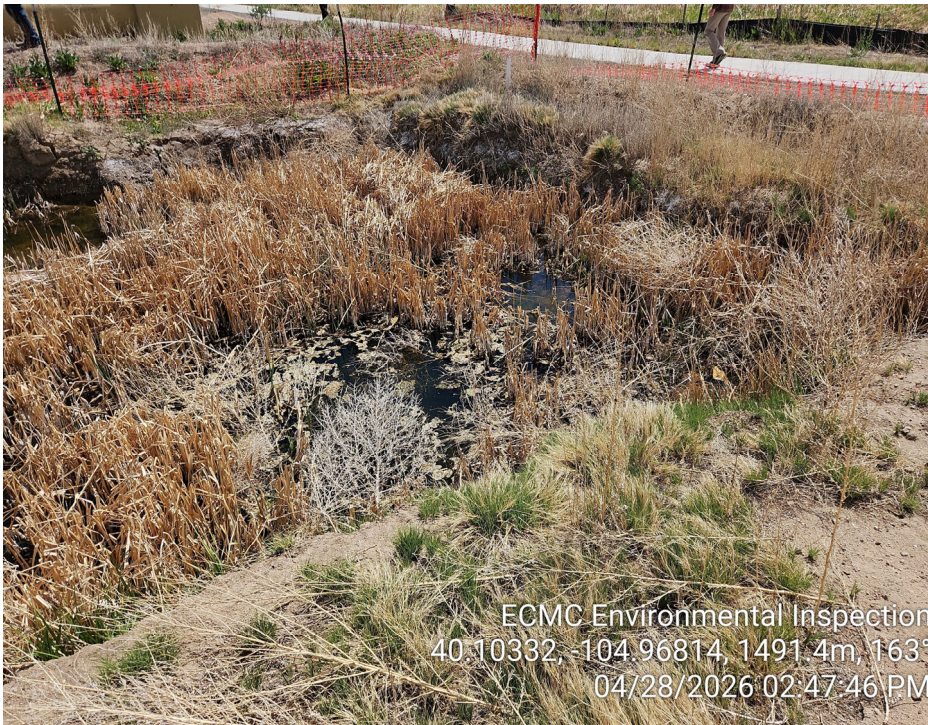
Photo 5 – Open excavation. Excavation visibility largely obscured by weeds. Groundwater present in open excavation.
