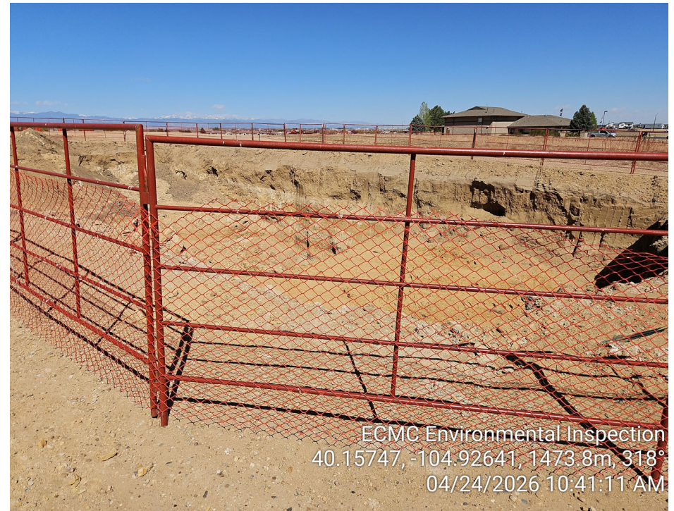
Photo 2 – Open excavation. Fencing adequate.
