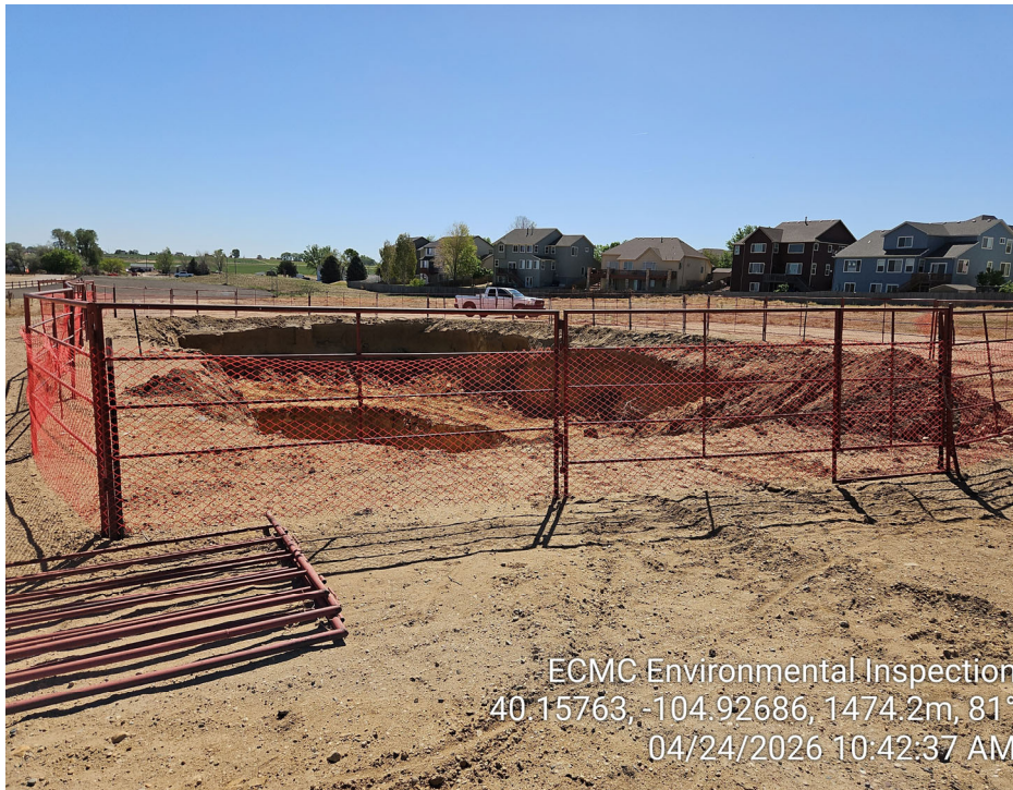
Photo 1 – Open excavation. Fencing adequate.
