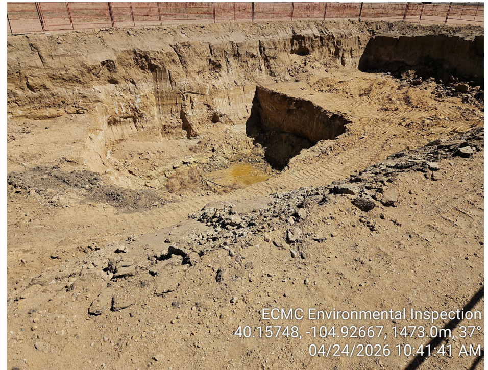
Photo 4 – Open excavation. Groundwater beginning to seep in.
