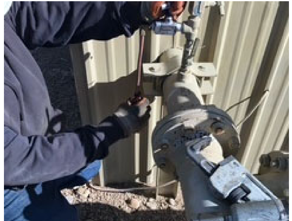
Attempted condensate sampling from Facility 5 Gas Sales Line – No condensate produced
