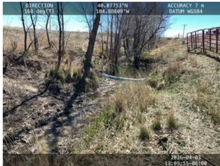
Hydrophobic oil-absorbent booms installed within Little Dry Creek adjacent to former excavation.
