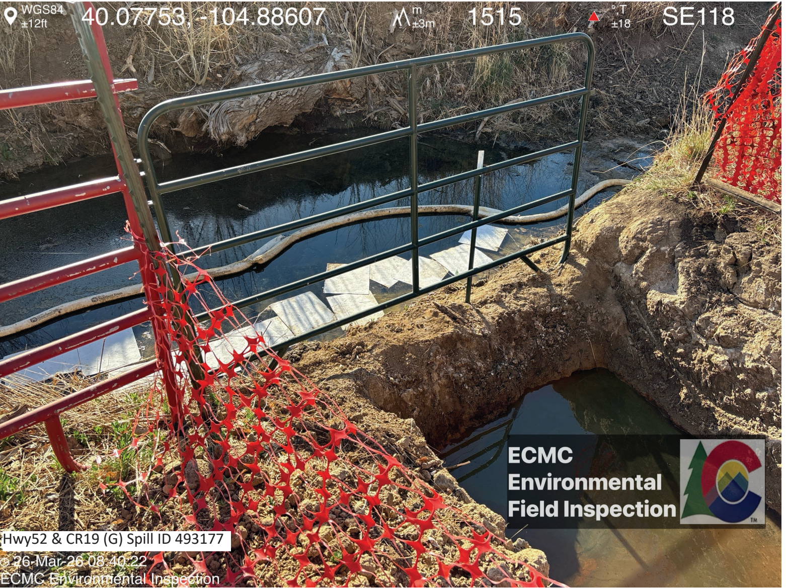
Hydrophobic oil-absorbent booms and mats placed in Little Dry Creek. A hydrocarbon sheen was observed on the surface of Little Dry Creek.
