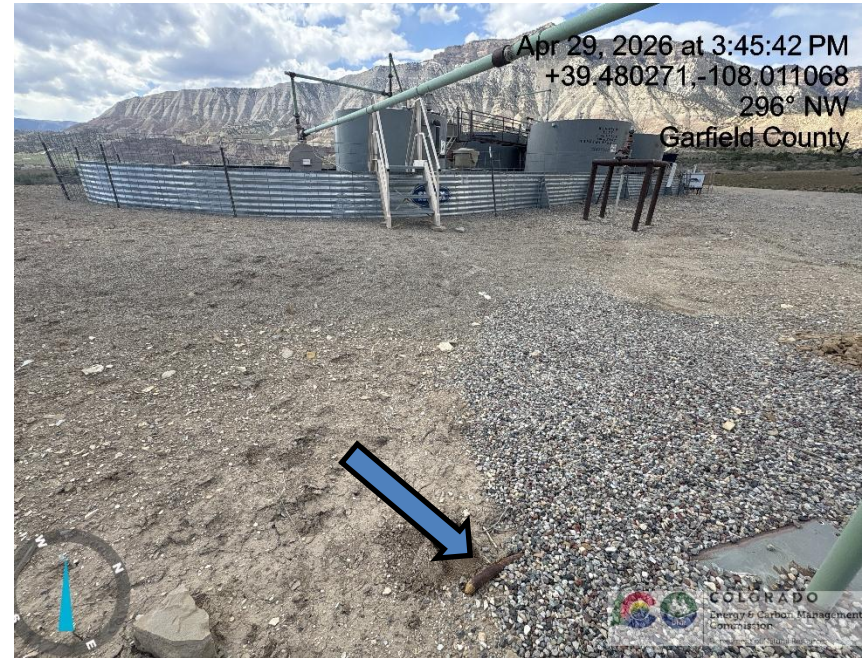
Photo # 4002 Same unmarked deadman
