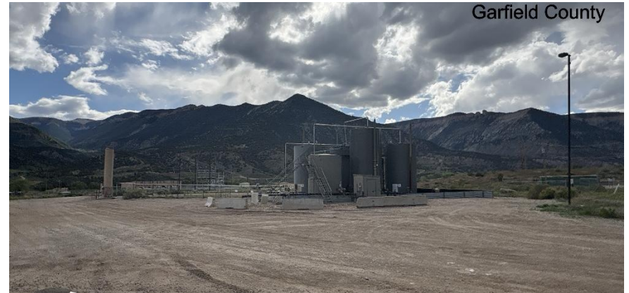
South East corner of location.
