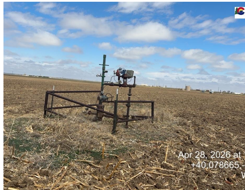
Pic 2 Wellhead sign missing on wellhead
