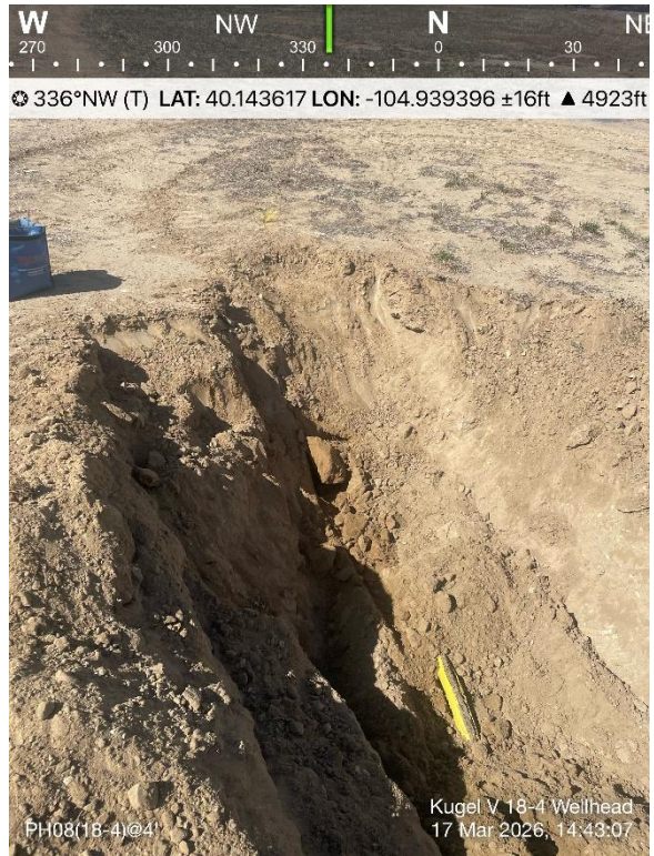
Flowline Pothole Screening Location 08
