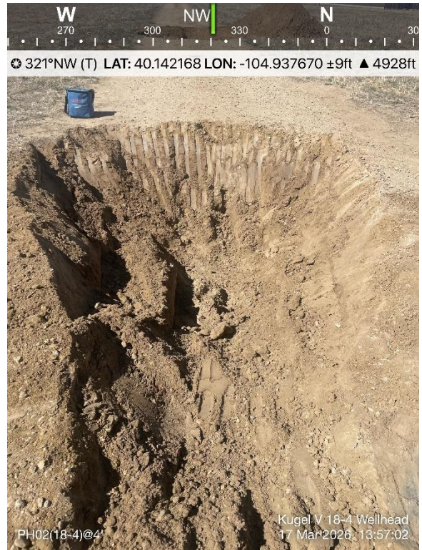
Flowline Pothole Screening Location 02
