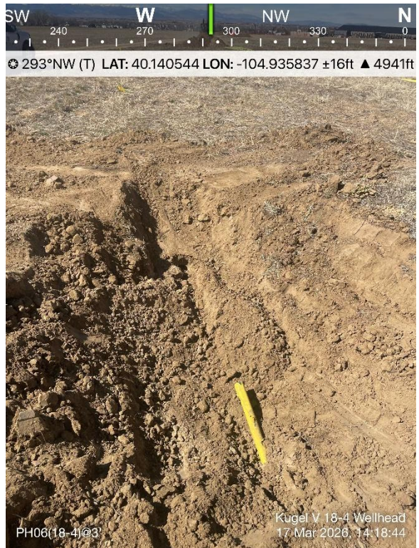
Flowline Pothole Screening Location 06
