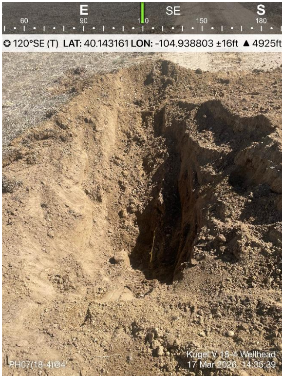
Flowline Pothole Screening Location 07
