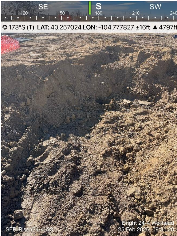
Separator Riser Sample Location
