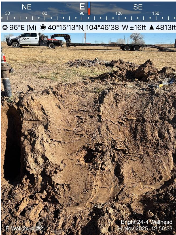
East Wall Screening Location
