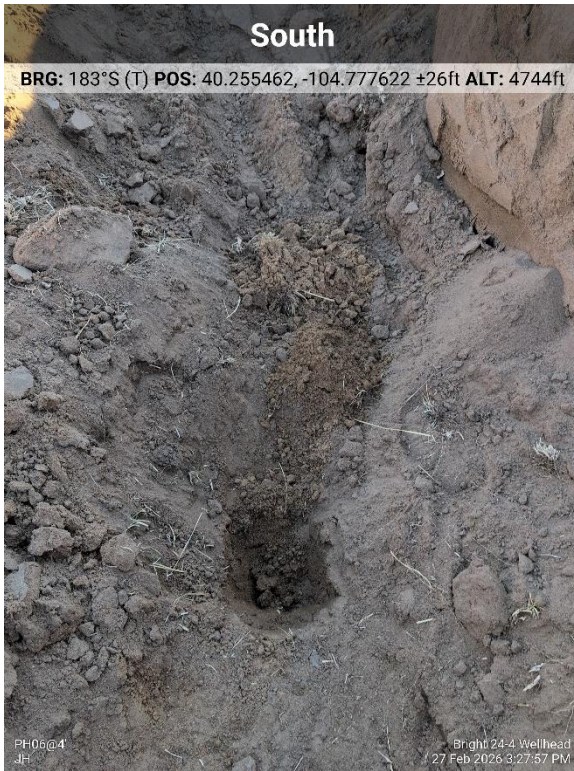
Flowline Pothole Screening Location 06
