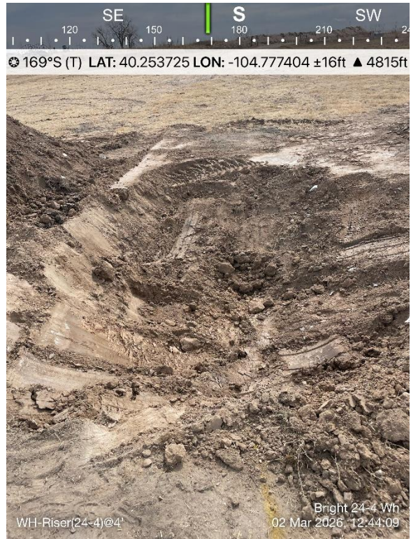
Wellhead Riser Sample Location
