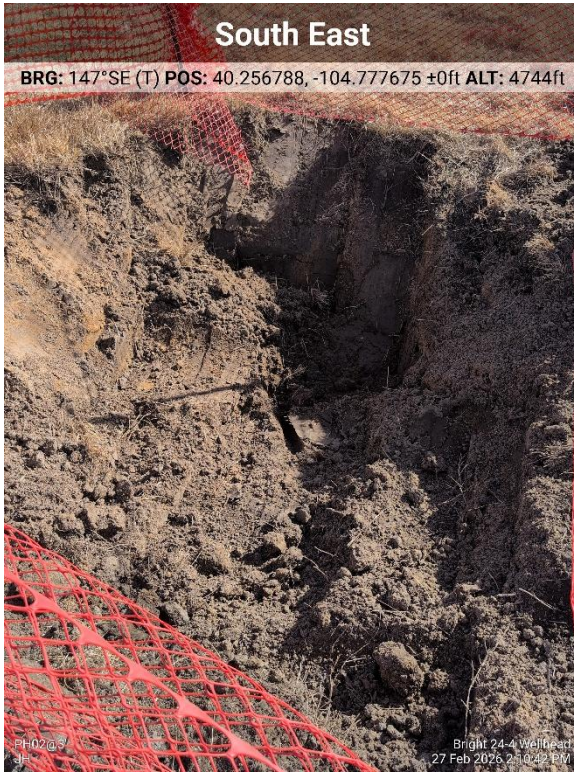
Flowline Pothole Screening Location 02
