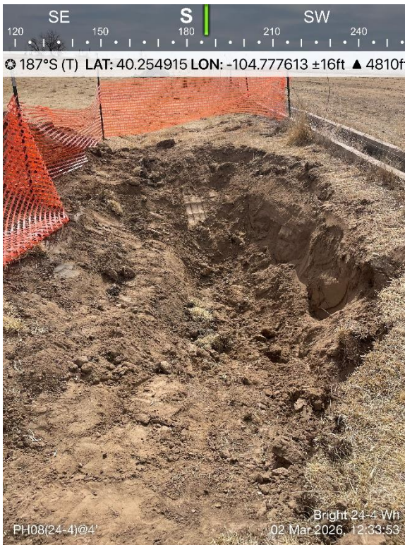
Flowline Pothole Screening Location 08
