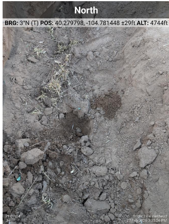
Flowline Pothole Screening Location 07
