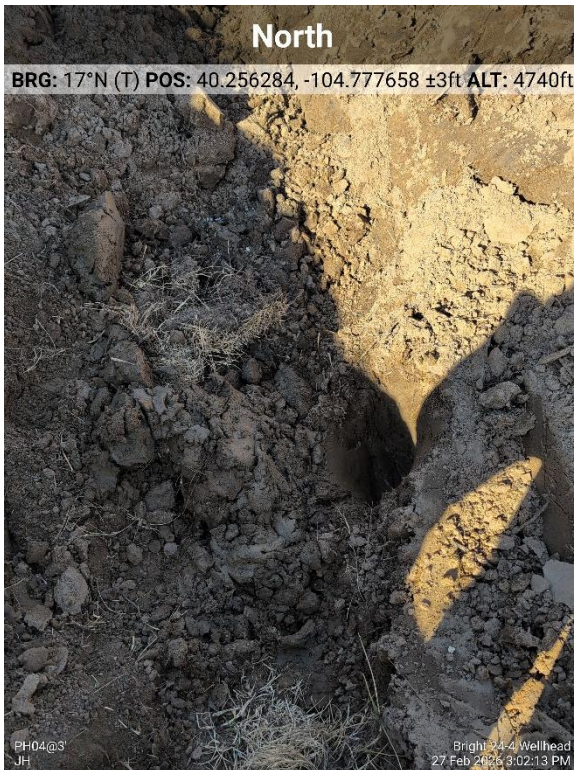
Flowline Pothole Screening Location 04
