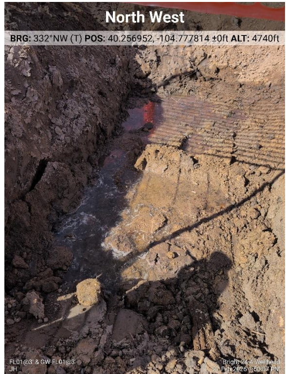
Flowline Pothole Soil and Groundwater Sample Location 01 (Groundwater Present)
