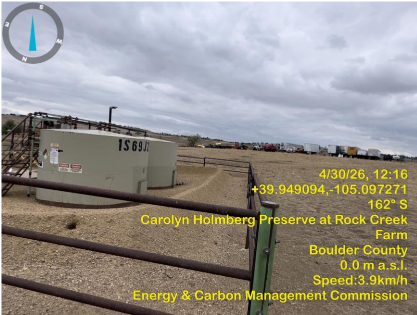
Photo 7 Tank battery.
