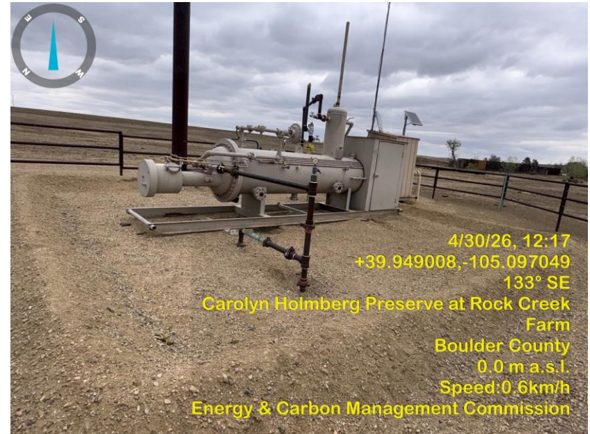
Photo 4 Horizontal Heated Separator LOTO.
