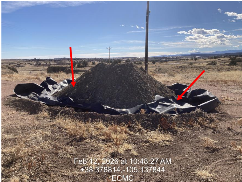
Photo 5 – Impacted spoil pile in containment
