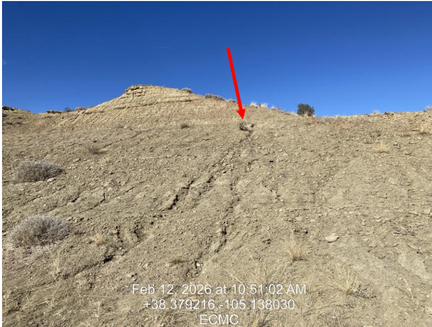
Photo 15 – Erosion on cut slope
