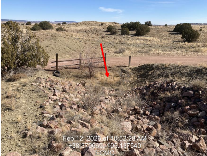
Photo 17 – Stormwater BMP adjacent to access Road is full
