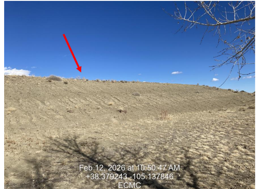
Photo 14 – Rilling along cut slope
