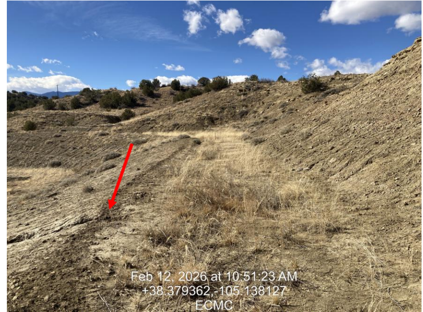
Photo 16 – Stormwater BMP at the top of cut slope is full, breach in dyke at red arrow
