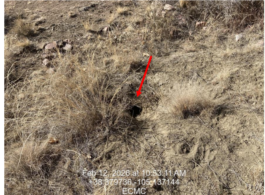
Photo 18 – Plugged culvert at lower end of BMP in photo # 17
