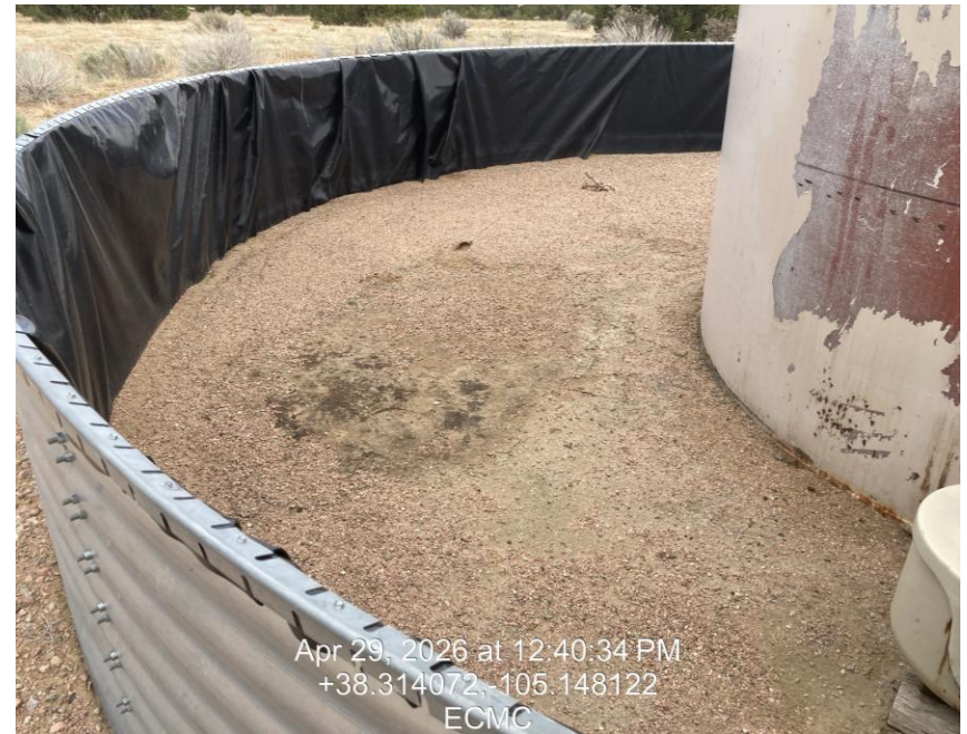
Photo 6: impacted material within secondary containment
