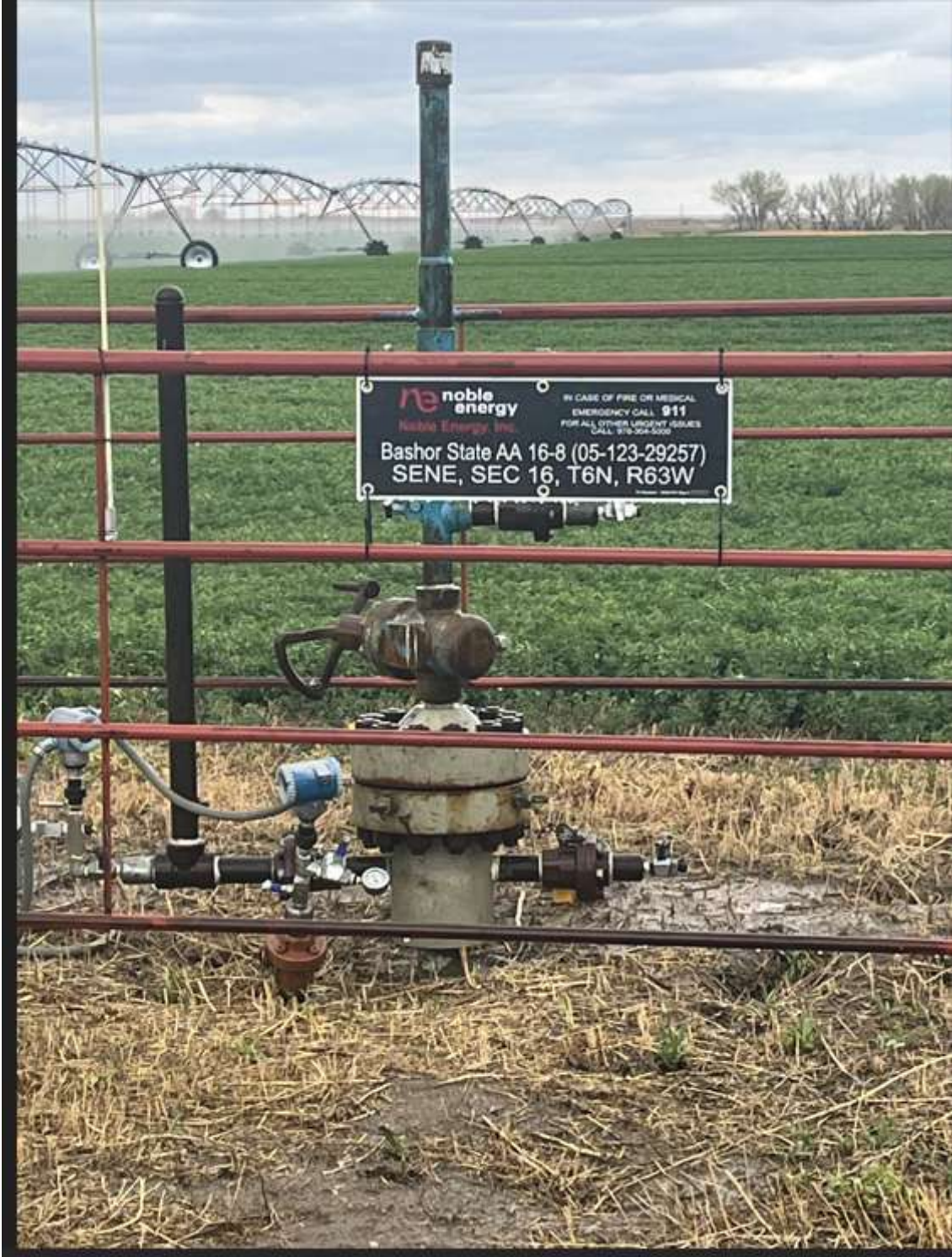
COMPLETION PHOTO - ECMC# 719700553 - BASHOR STATE AA 16-08, WELL
