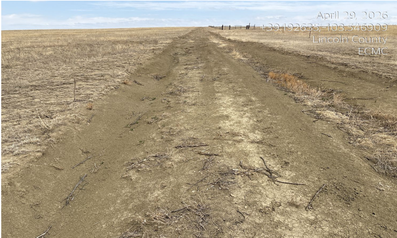
Photo 2. Facing north along the pre-existing road.
