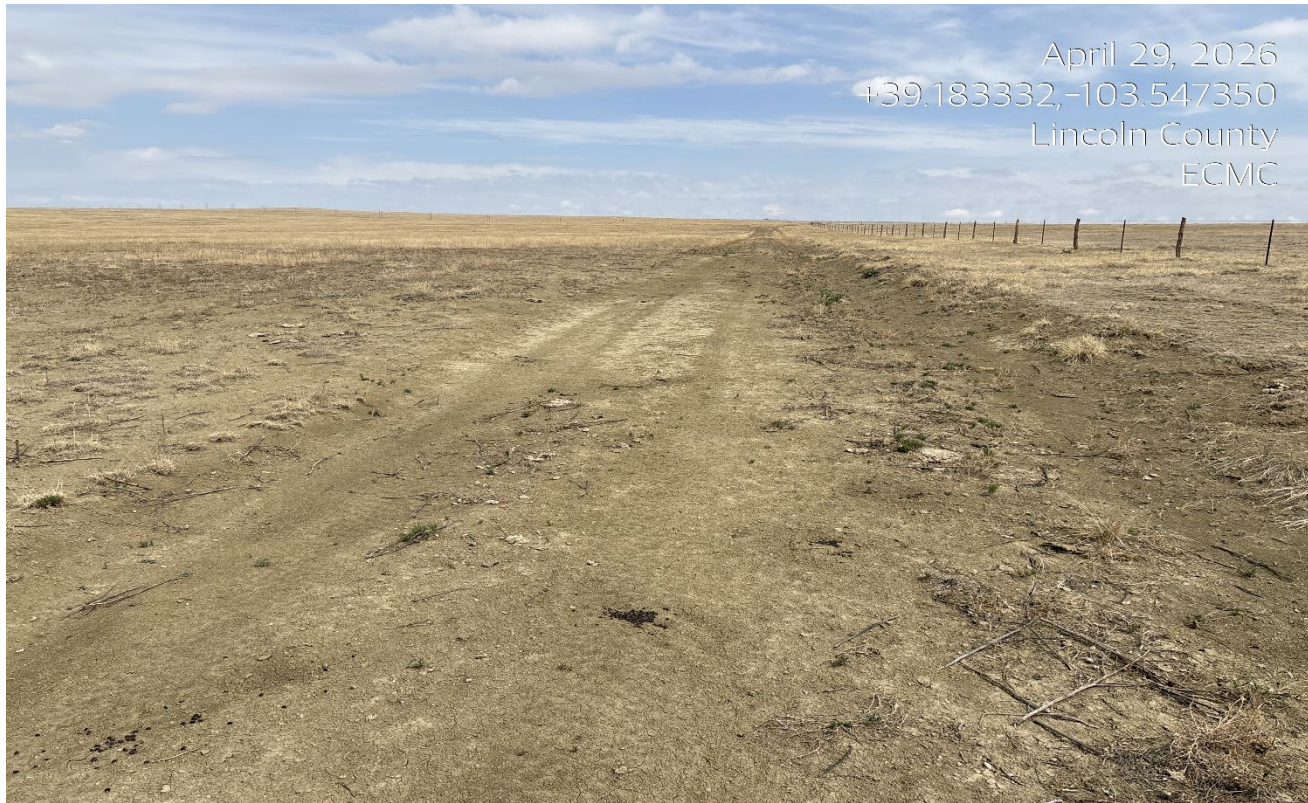
Photo 1. Facing north along the pre-existing road. It appears this road has been graded since the previous inspection.
