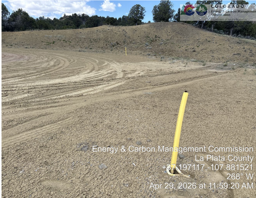
11. Rig anchor markers on north end.
