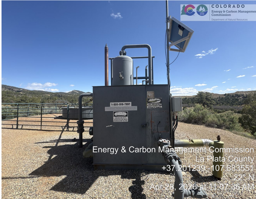
11. Vertical heated separator/meter run combination. Meter calibration card displayed inside door on right side inside plastic sleeve. Dated 07/07/2023. Labelled “Chevron Midstream” not “Enduring Resources”.
