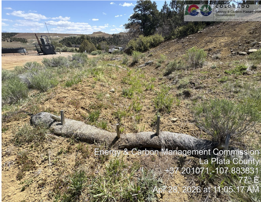
19. Straw wattles in southern reclamation area run-on diversion ditch are full of sediment.
