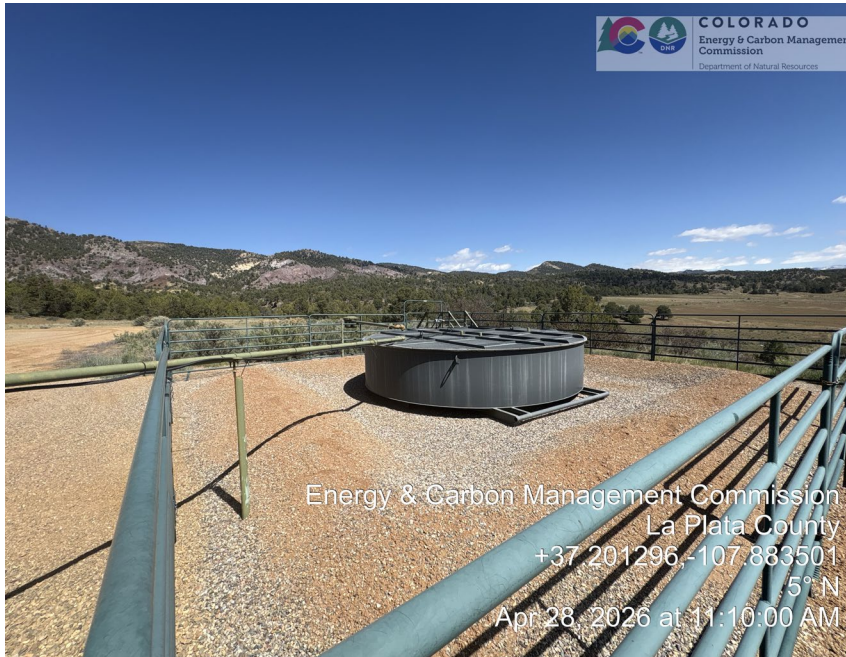
13. Open topped steel produced water tank from SE Corner. Lat Long = 37.201296/-107.863501. Berm appears to be adequate.
