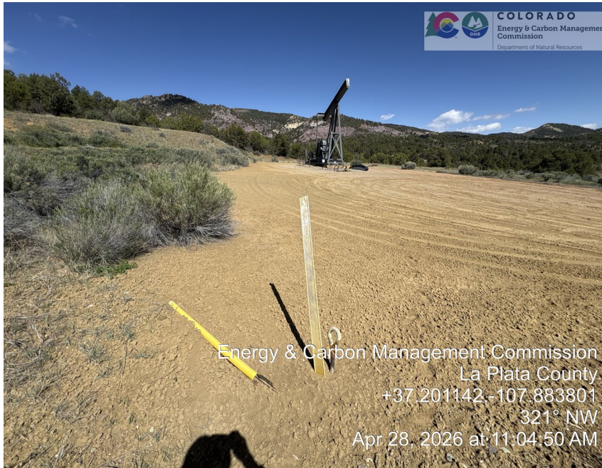
17. Overview of well pad from SE corner looking NW. Rig anchor marker is down. Also marked with "Gas Pipeline" fiberglass marker.
