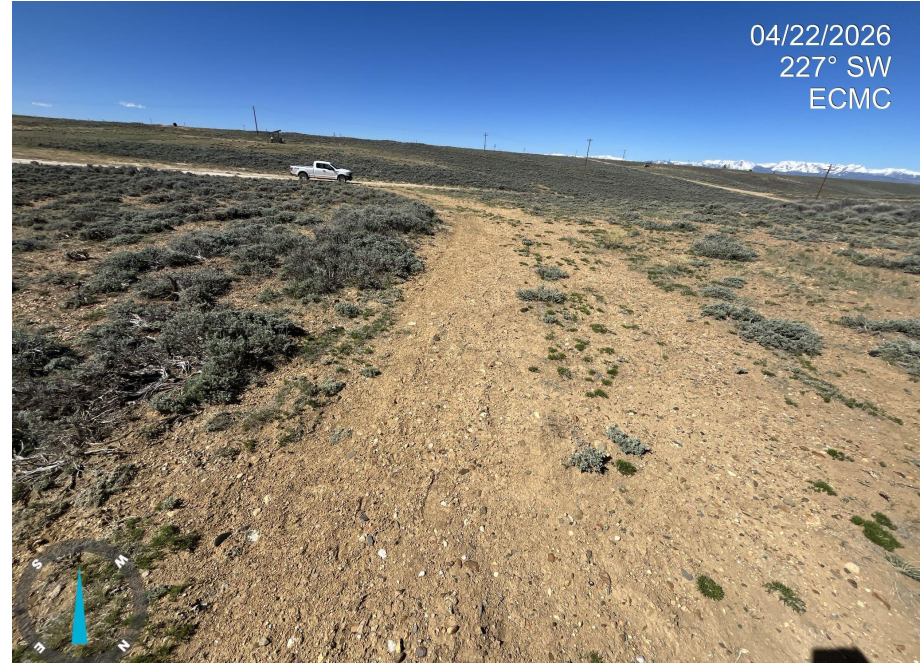
Photo 10. Photo illustrates that the access road has not been reclaimed.
