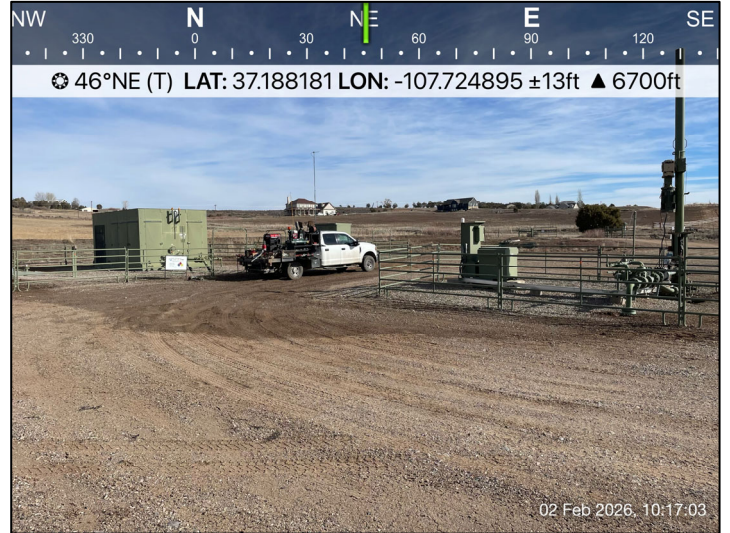
Photograph: 2 Description: Release area
