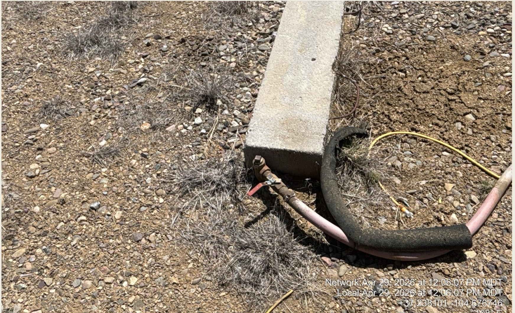
PHOTO 5: UNUSED EQUIPMENT (1" RISER NOT IN USE OR USEFUL). REMOVE OR IDENTIFY THE CONTENTS PER RULE 606. CA DATE 5/29/2026.
