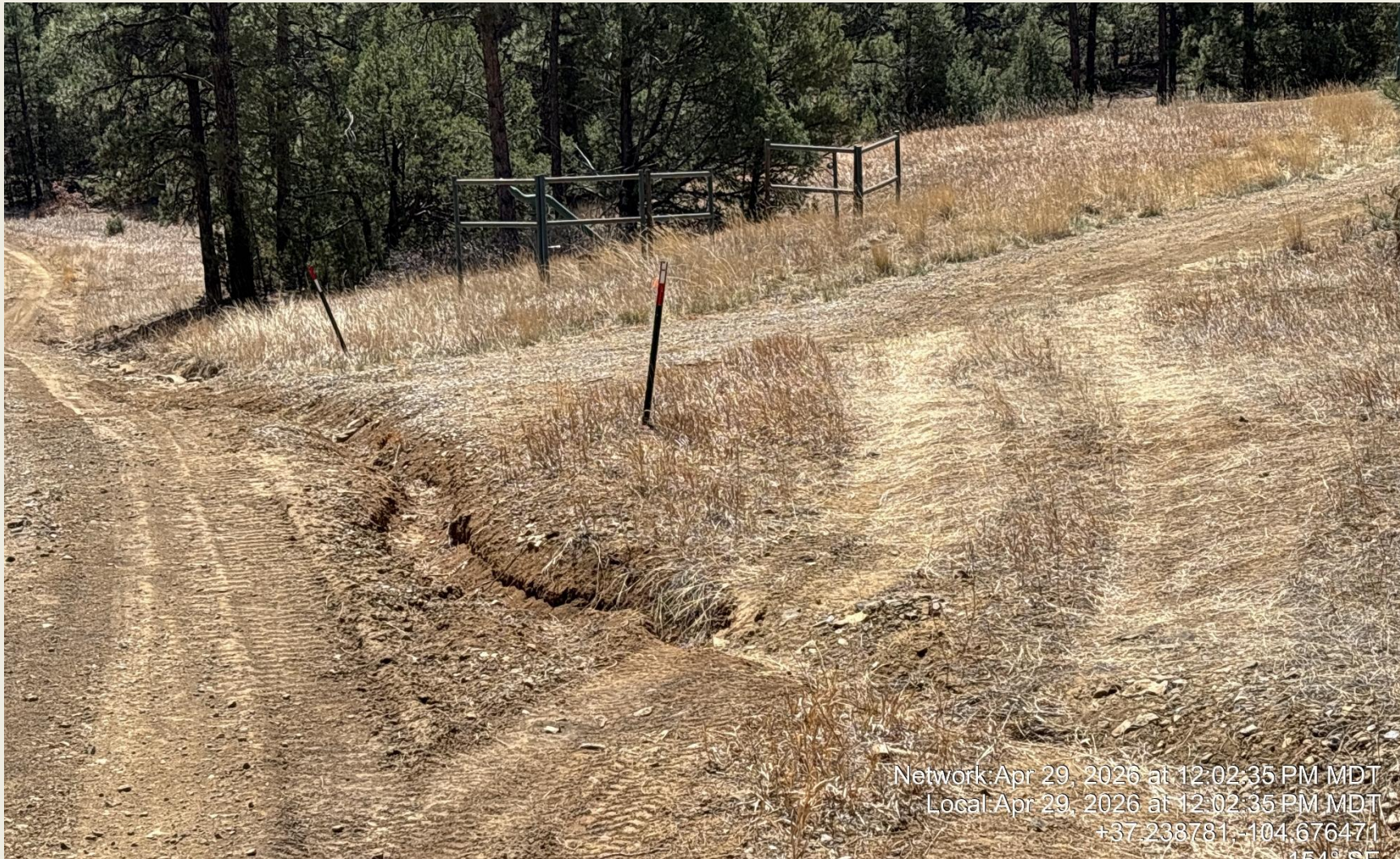
PHOTO 7: STORMWATER EROSION AT ENTRANCE OF LOCATION VEHICLES ARE DRIVING OFF OF THE ROW TO BYPASS THE EROSION. IMMEDIATELY STOP ALL VEHICLES FROM DRIVING OFF OF THE ROW AND INSTALL BMP'S TO PREVENT STORMWATER EROSION FROM DAMAGING THE ROW PER RULE 1002. CA DATE 5/5/2026.
