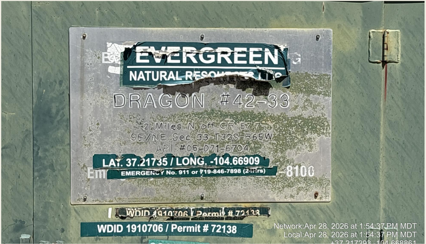
PHOTO 2: WELL SIGN IS NOT LEGIBLE FROM A DISTANCE (NEW SIGN IS STORED INSIDE METER HOUSE). REPLACE SIGN PER RULE 605. CA DATE 4/30/2026.
