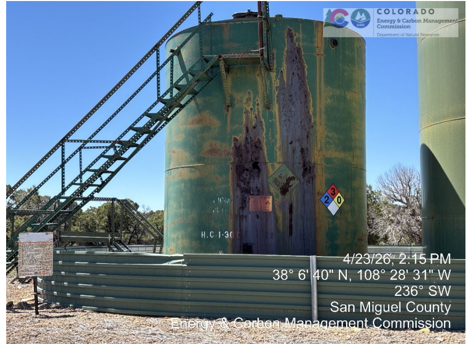
Tank with rust holes
