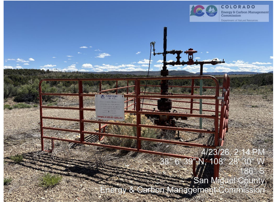
Wellhead with fence and sign
