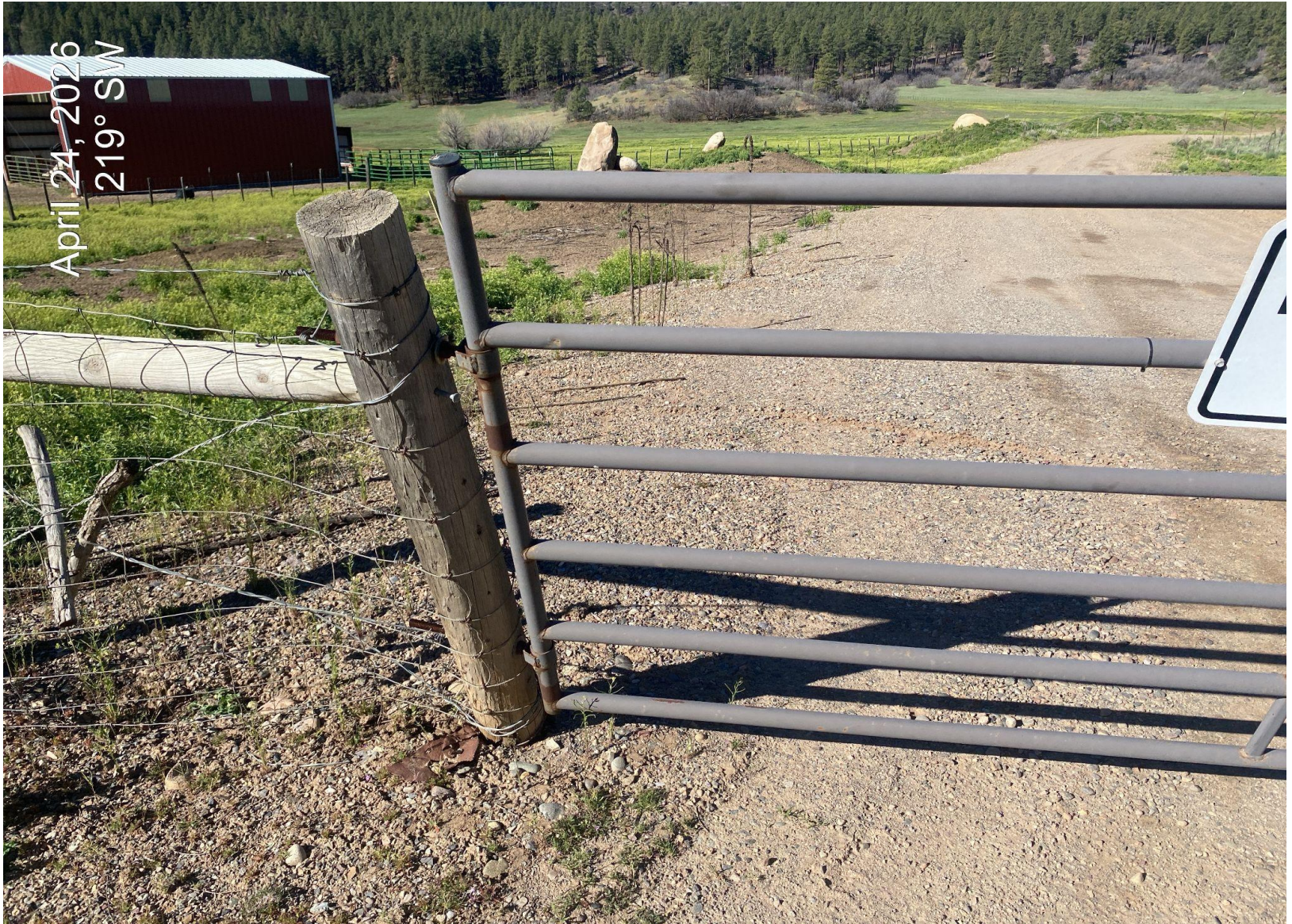
Photo 4. Access point gate pole is rotting and beginning to fall.
