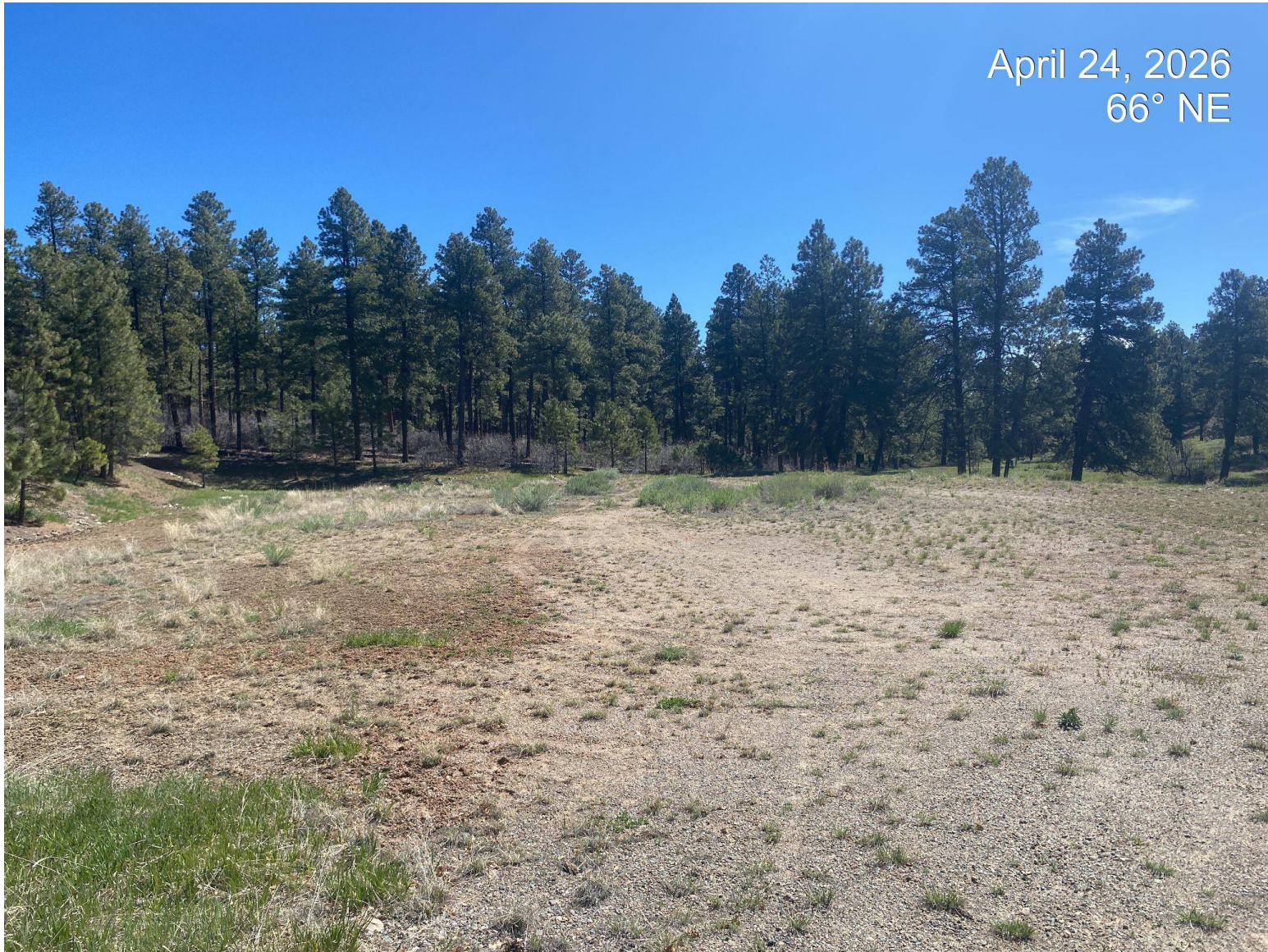
Photo 3. View of well pad; surface equipment has been removed but pad remains unreclaimed with gravel and has not been recontoured.
