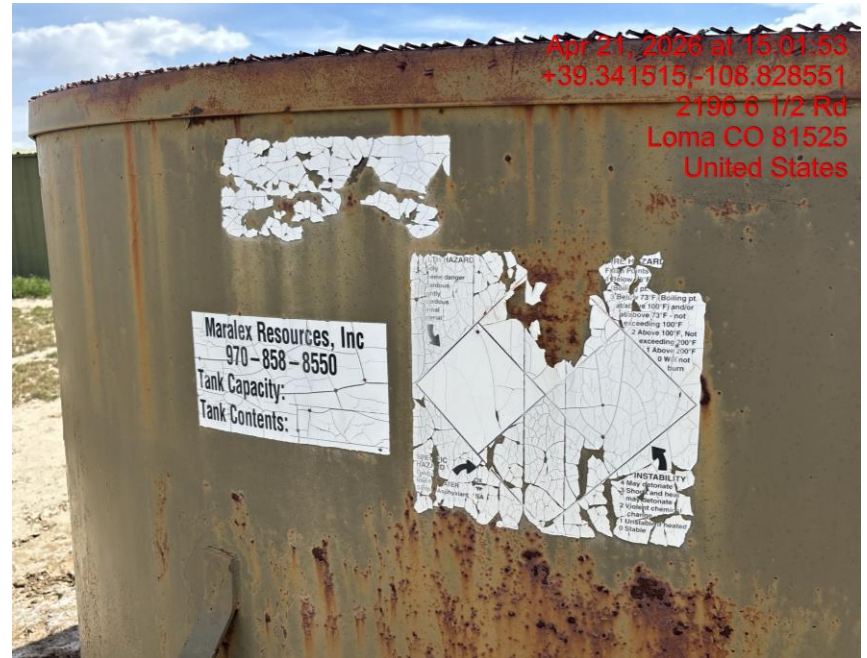
Unserviceable Tank Labeling – Photo #03582
