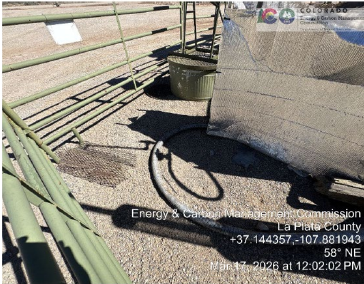
43. Unused expanded metal machinery guard at 36-1A
