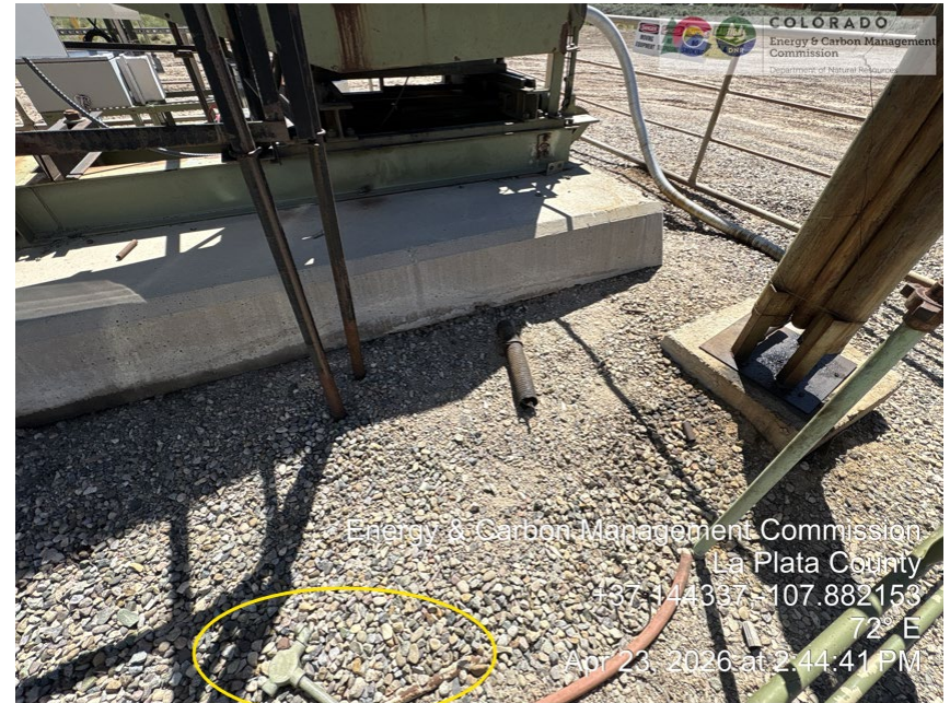
30. After. Conduit and wires remain on ground. Different angle. Same conduit in yellow circle.
