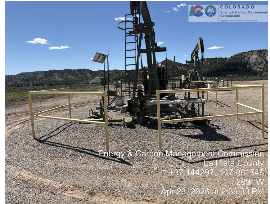
34. After. Leakage appears to have stopped. Photo 49 of this report is a zoomed and cropped version of this photo that shows better detail.
