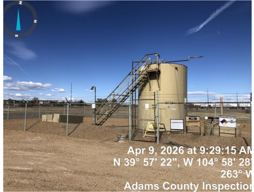
PHOTO#2 PRODUCTION TANKS
