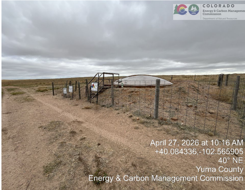
Tank and signs
