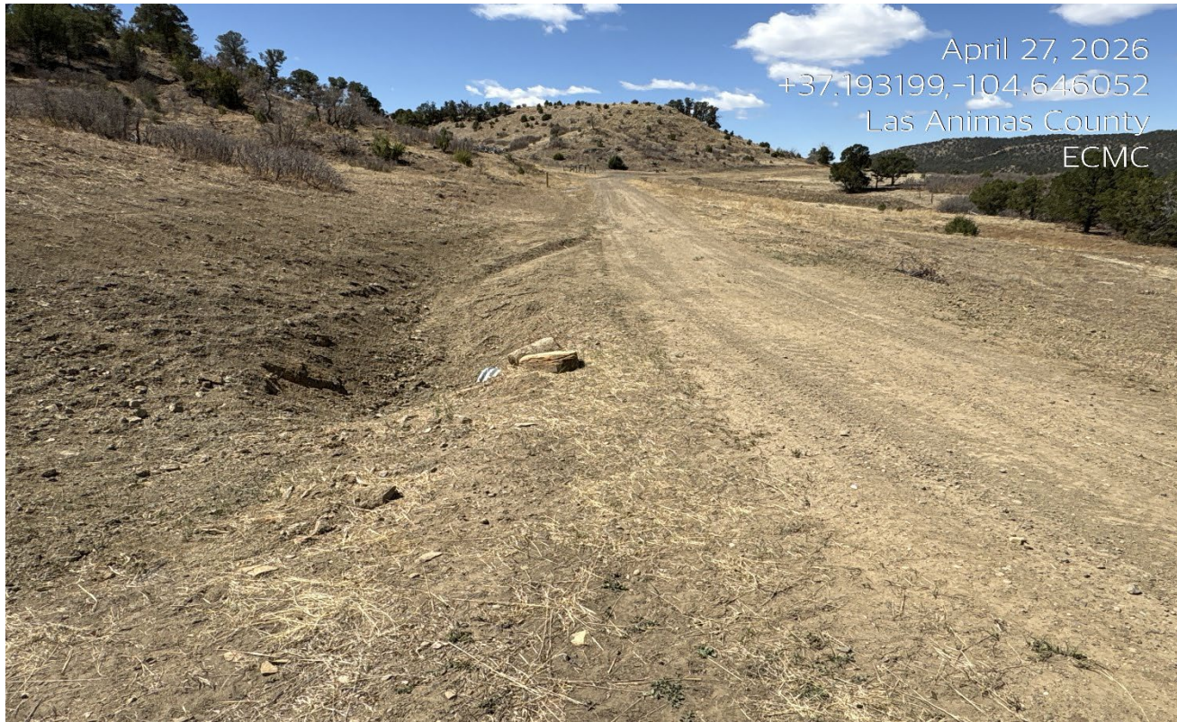
Photo 1. Facing south along the access road. The culverts are cleaned out and maintained.
