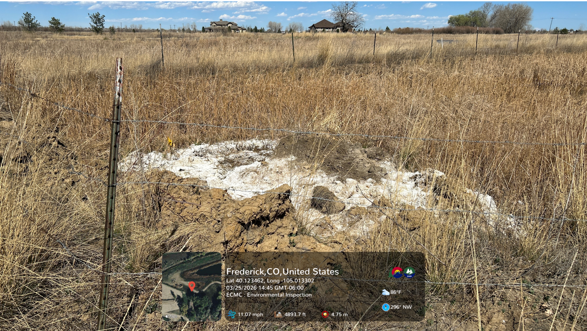
Salt crusting is visible within the excavation.
