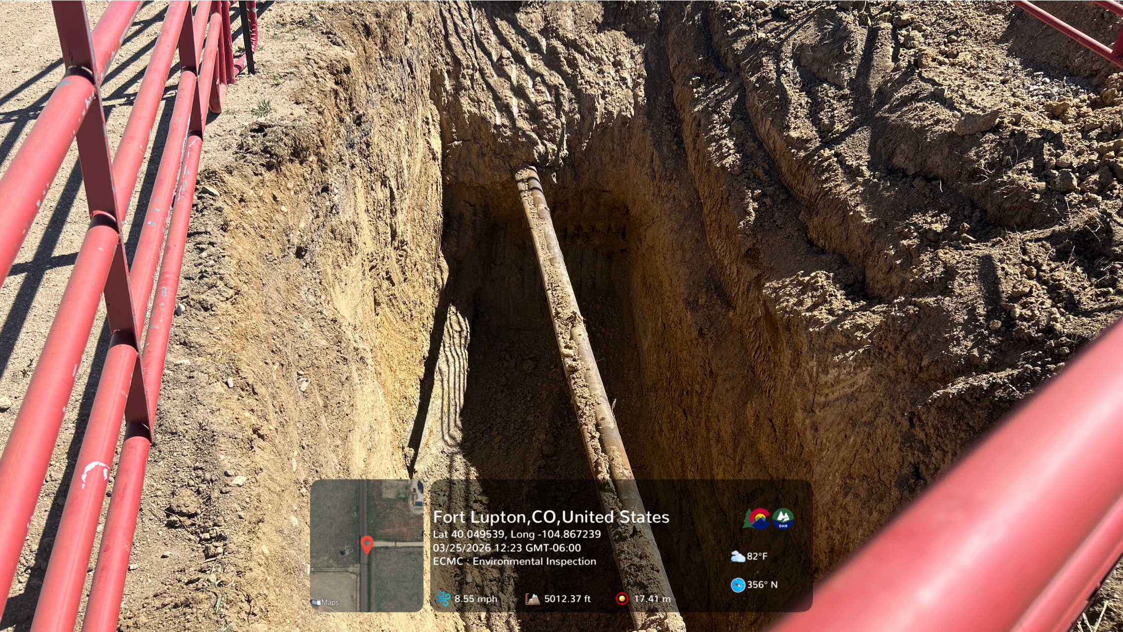
Flowlines are visible in the open excavation.
