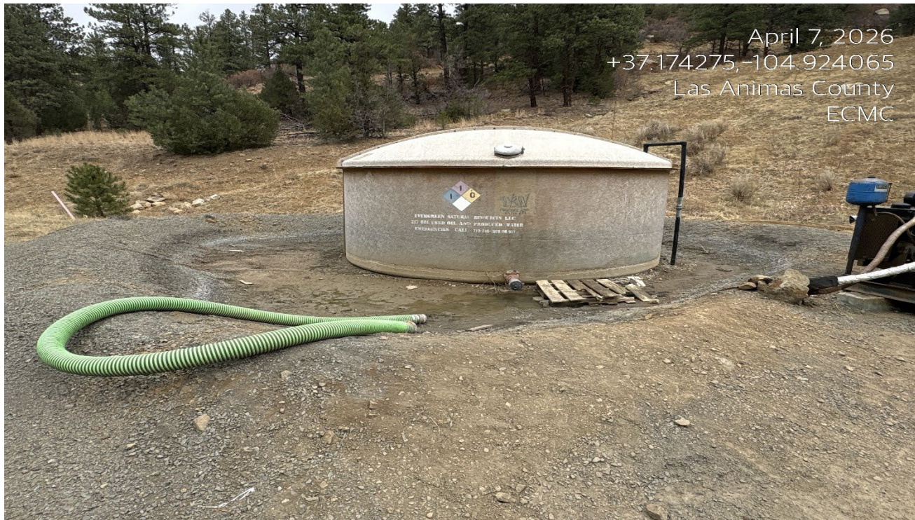
Photo 3. There was wet soils and a dripping leak at the tank which was inside secondary containment.
