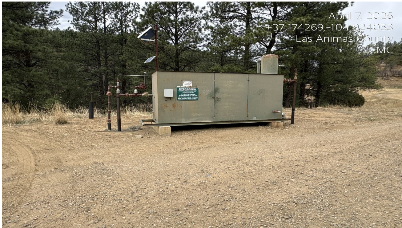
Photo 1. Well sign posted at meter shed.
