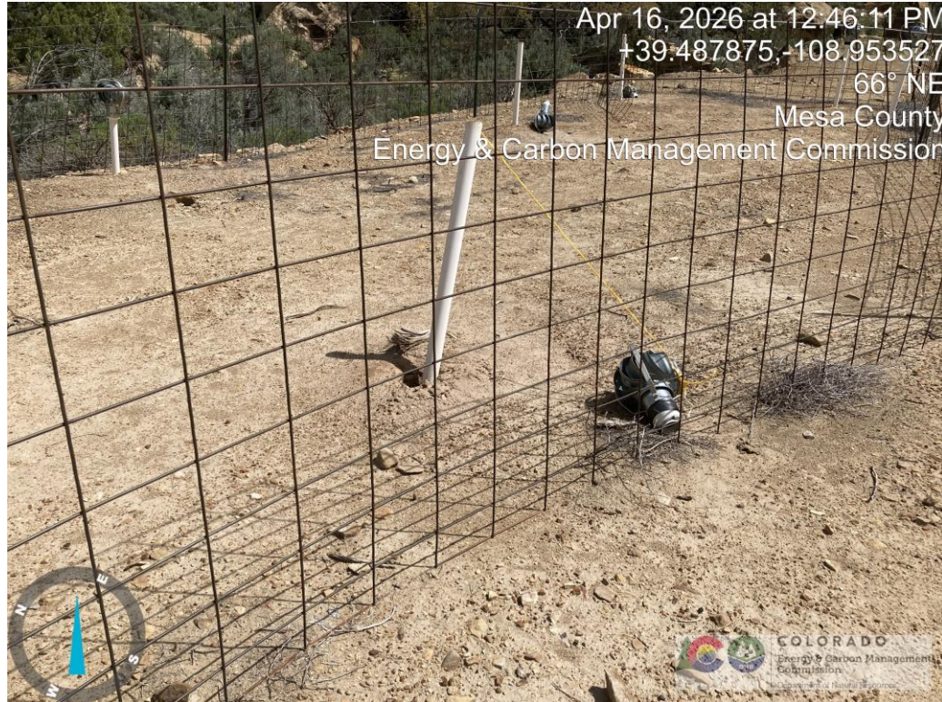
Turbine off of vent.
