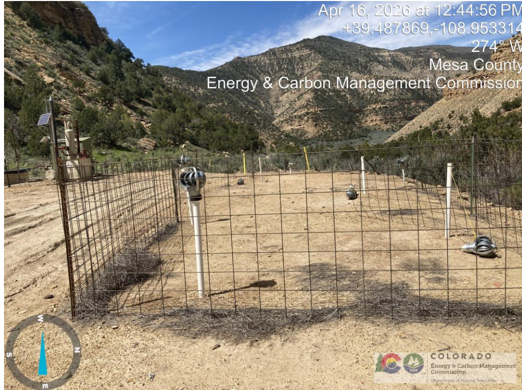
Turbines are off 3 of the 7 vents.
