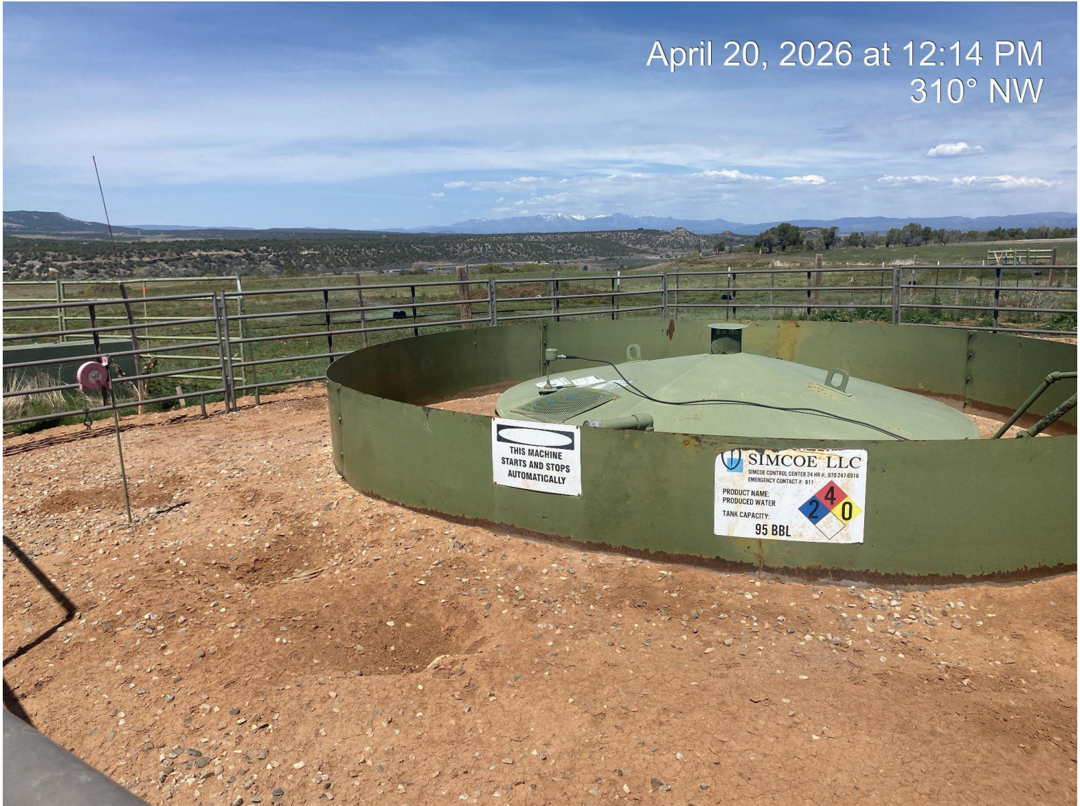
Photo 2. Secondary containment ring installed around produced water tank.
