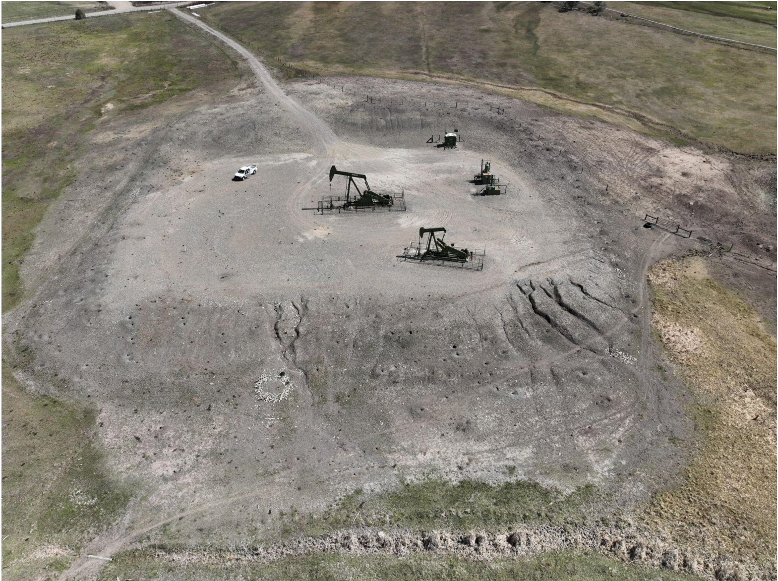
Photo 4. Drone aerial of the location. Note: Location does not meet interim reclamation vegetation standards and active erosion occurring on southern edge of location.
